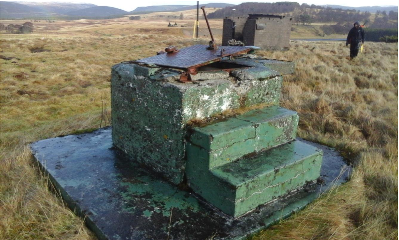
Plate 5. Area 3 looking north east showing the bunker and aircraft post
