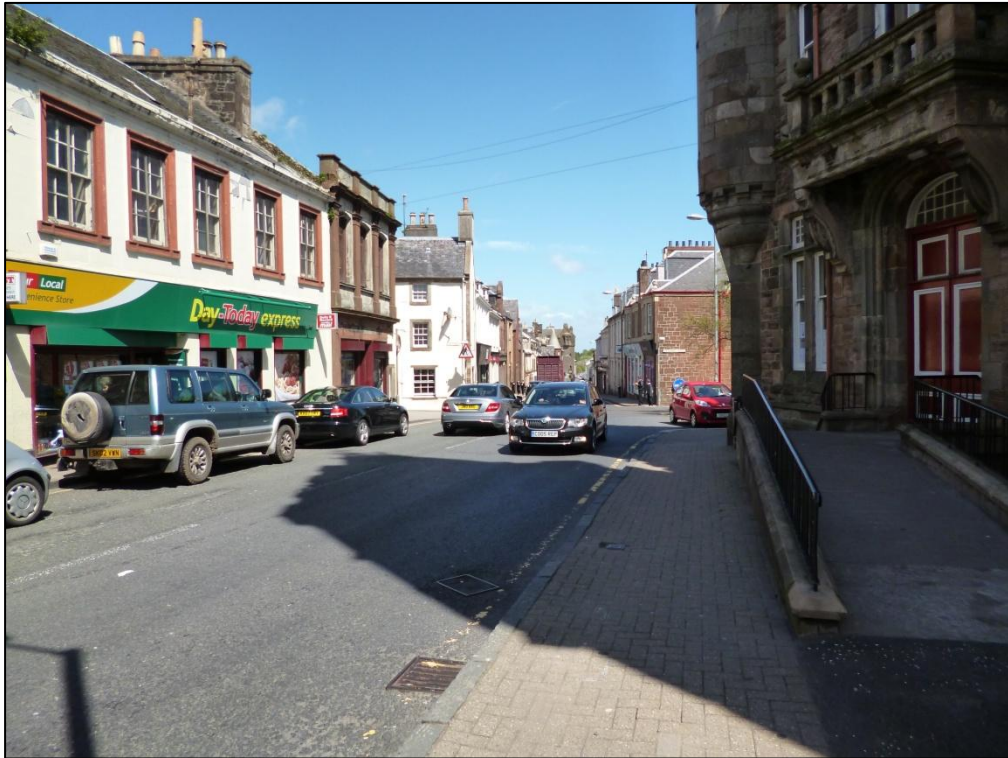
Figure 11.1. Conditions on the existing A77 through Maybole town centre
