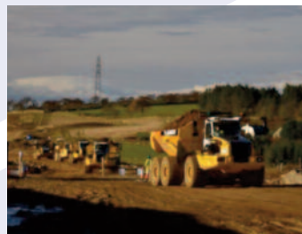
The long haul begins in the Central Section
