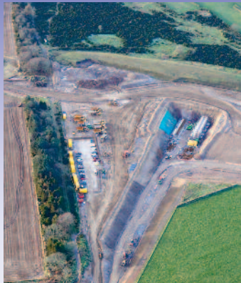
North Kingswells Junction Underbridge
