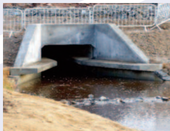
Culvert 41 North Section
