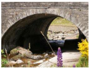
Figure C.43 – Old Masonry Bridge extended to form large culvert NGR location NN640730
