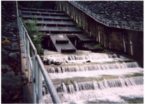
Figure 8.13 – Detail of a concrete spillway on the downstream face of a debris basin barrier, Harvey Creek, Sea-to-Sky Highway, British Columbia, Canada. The drainage outlet may be seen in the centre of the spillway.
