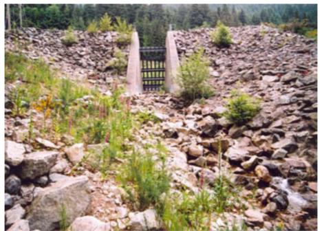
Figure 8.10 – Debris basin showing the downstream barrier and drainage outlet, Mackay Creek, North Vancouver, British Columbia, Canada.
