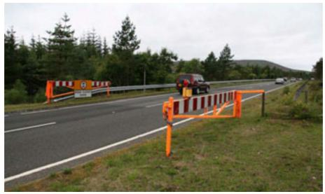
Figure 8.1 – Snow gates on the A9. These are used to close the road over Drumochter Pass when it is impassable due to snowfall. These and similar installations could also be used to close the road in the event of debris flow.
