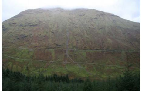
Figure 2.14 – View of the hillside above and below the approach from the east to the Rest and be Thankful (from NGR NN 23160 06559 on the opposite side of Glen Croe). Not only can the event dated 28 October 2007 be clearly seen but evidence of numerous past events can be seen on the surrounding hillside.
