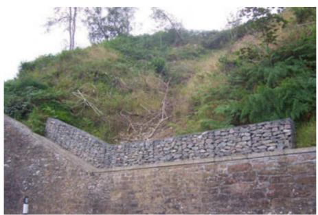
Figure 2.28 – Gabion debris trap, Struie.
