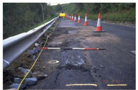
Figure 8.23 – Deformation of the A86 carriageway alongside Loch Laggan due to a series of minor landslides.
