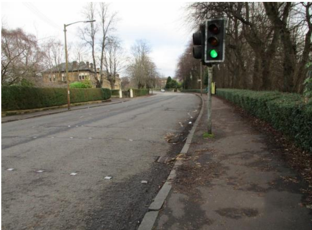
Figure 5: St Andrews Drive, pre-construction.
