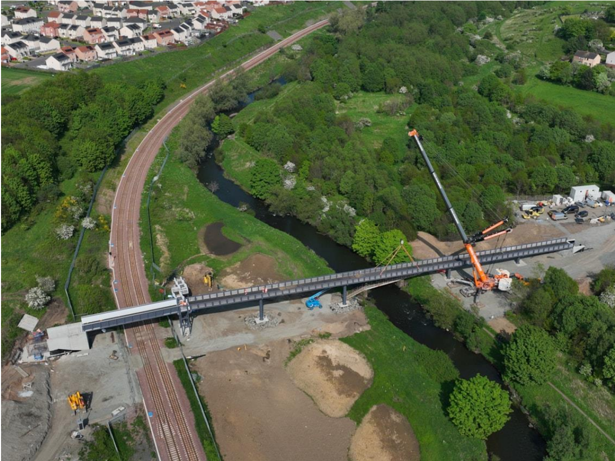
Figure 15: Installation of the new Duniface footbridge.
