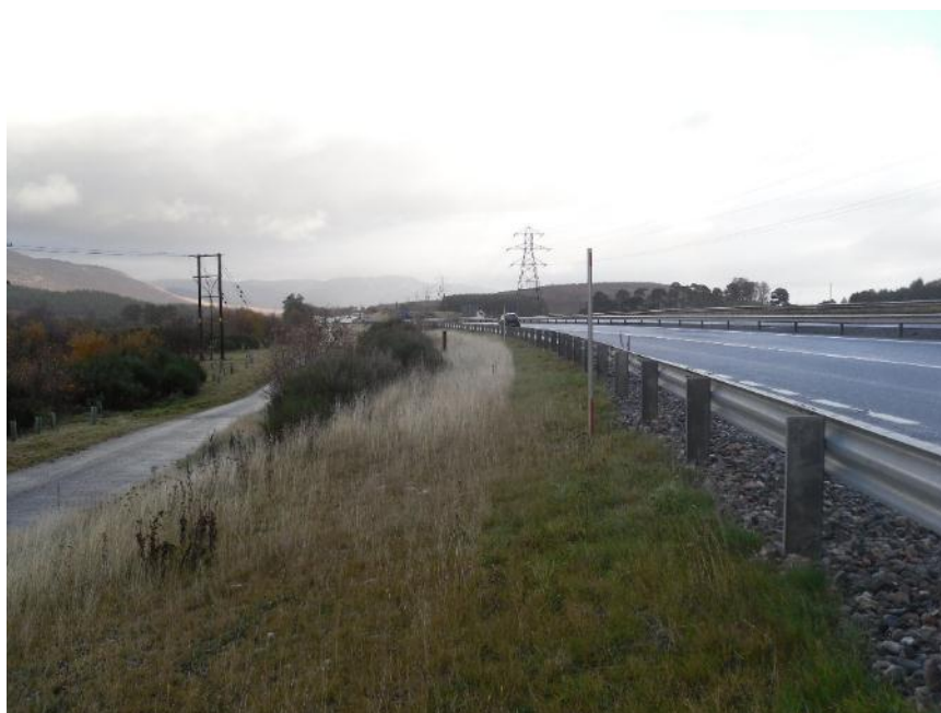
Figure 7 Grass along the northbound carriageway
