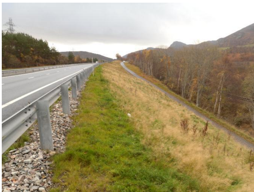
Figure 12 Regeneration of area adjacent to cycle path
