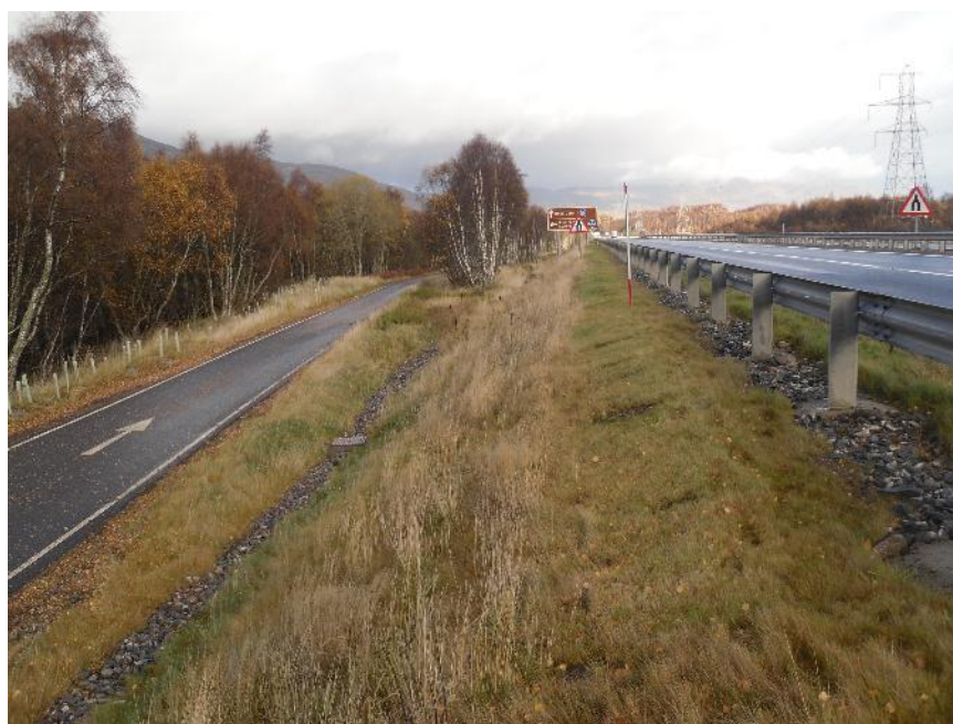
Figure 13 Existing cycle path retained as part of scheme
