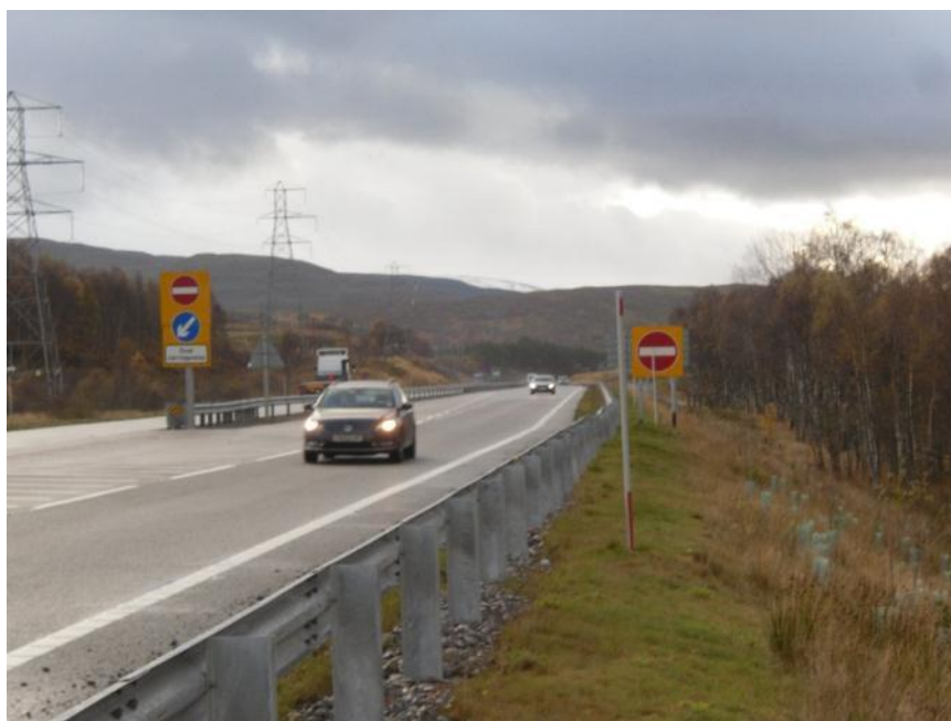
Figure 1 Northbound carriageway looking South
