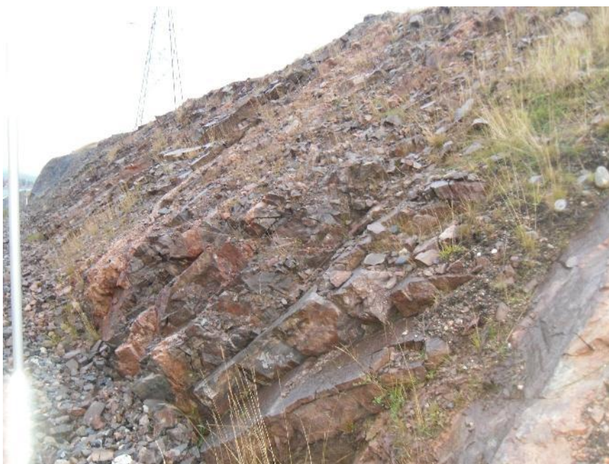
Figure 10 Evidence of grass growing on newly exposed rock face
