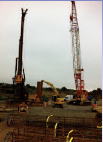
Piling works adjacent to the River Dee
