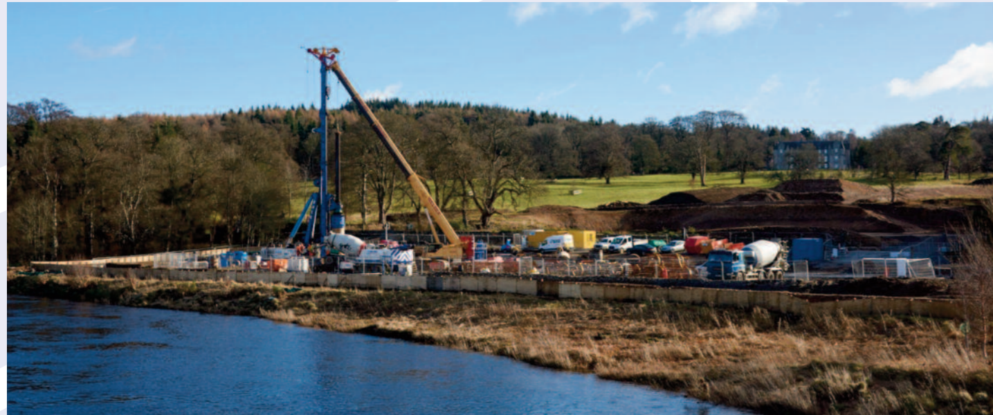
Piling works at the River Dee crossing
