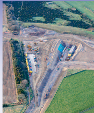
North Kingswells Junction Underbridge
