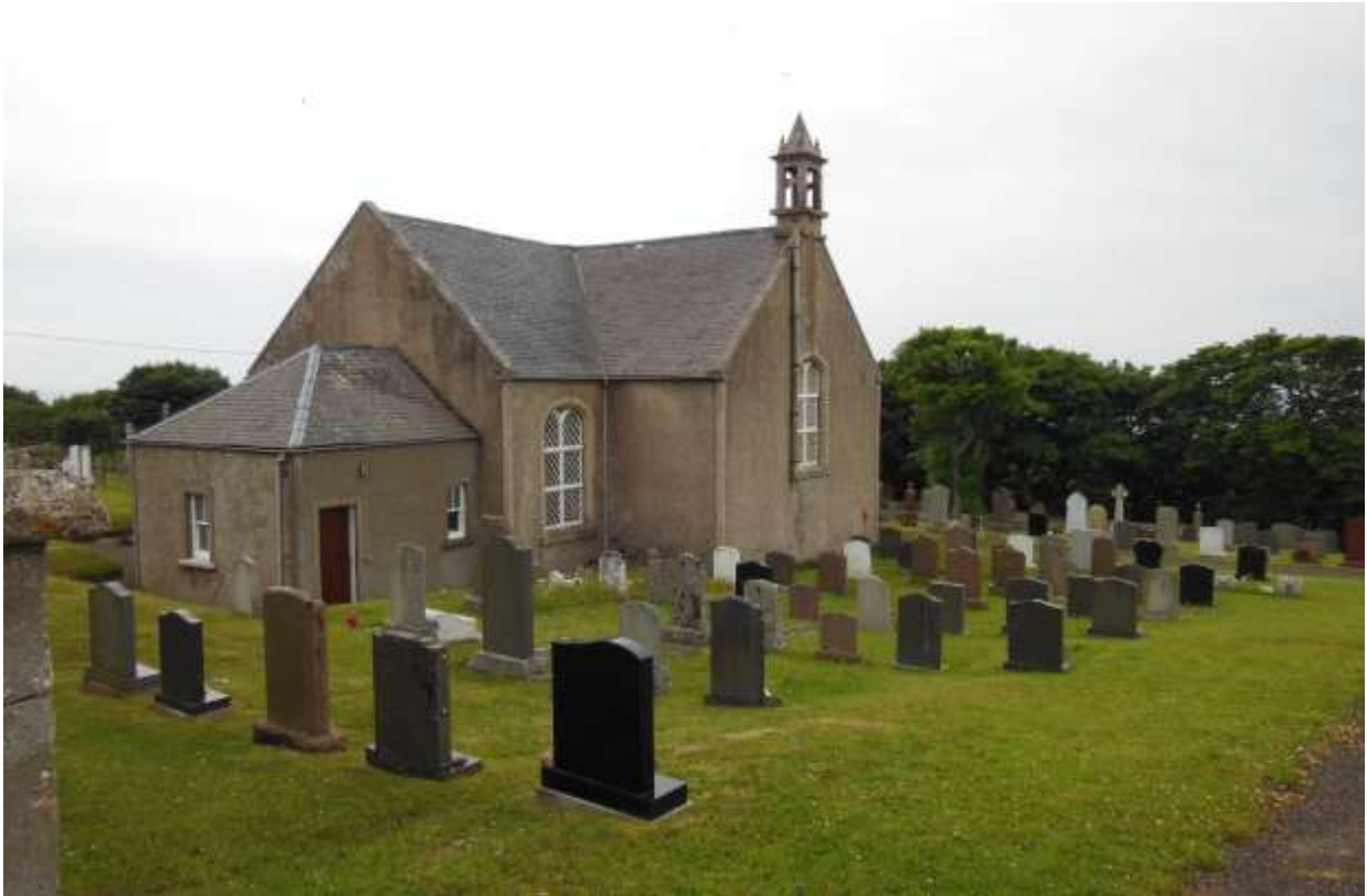
Plate 8 Berriedale Parish Church looking southwest
