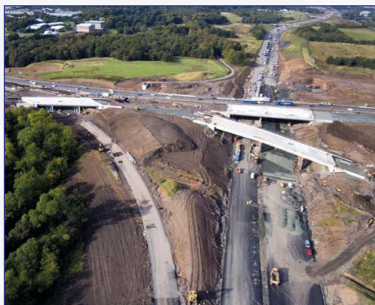
Progress at Shawhead Junction
