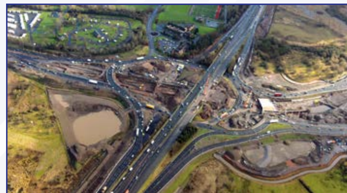
Construction Progress At Raith
