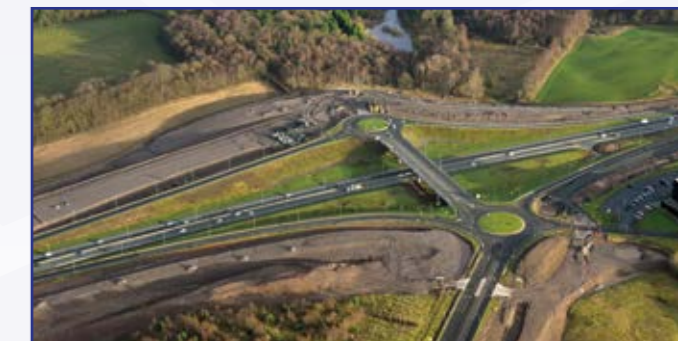
Excavated earth has been reused at Eurocentral
