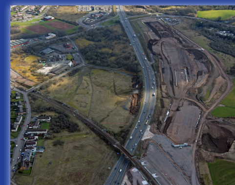
New M8 south of A8, Bargeddie
