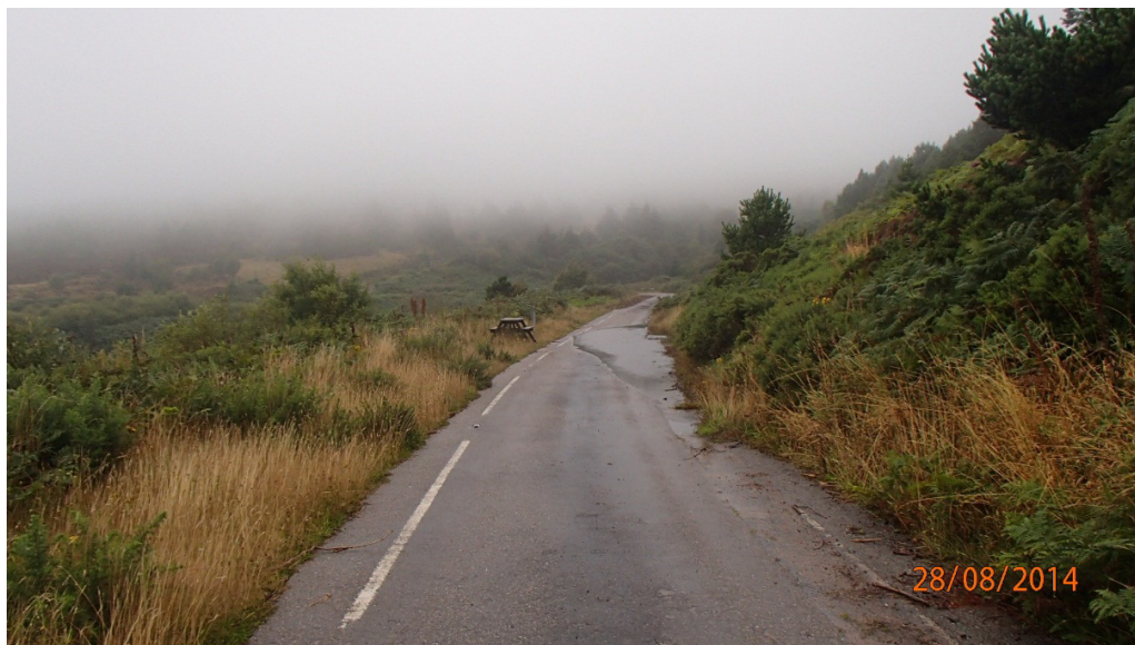
Figure 10: Remnant road markings and road studs from old A9 left in situ at picnic area viewpoint
