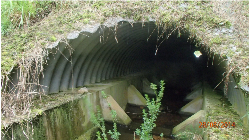
Figure 8: Culvert with otter ledges and fish pass
