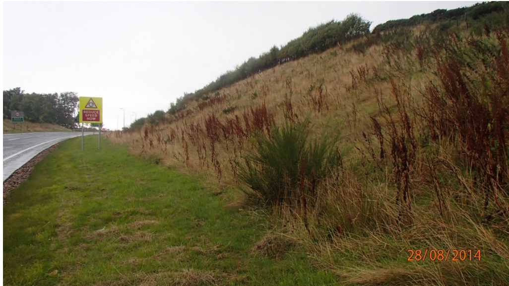
Figure 4: Natural regeneration on embankment with areas of dock and nettles
