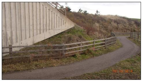
Figure A.3: Missing section of the mammal fence by the underpass at Bellyford Burn
