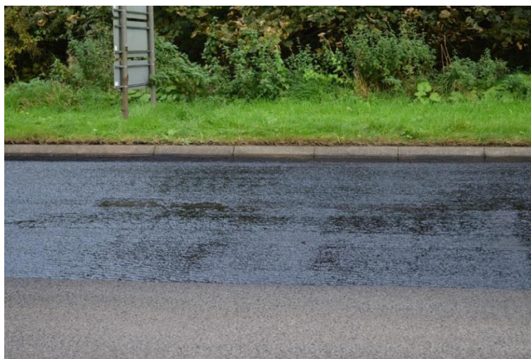
Figure C-5 Tack coat prior to surfacing
