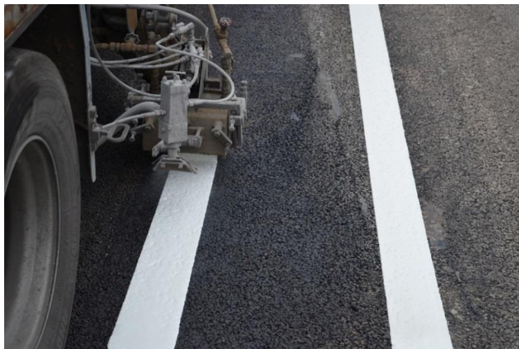
Figure C-8 Line marking application
