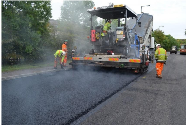
Figure C-1 Construction of asphalt surfacing (TS2010)
