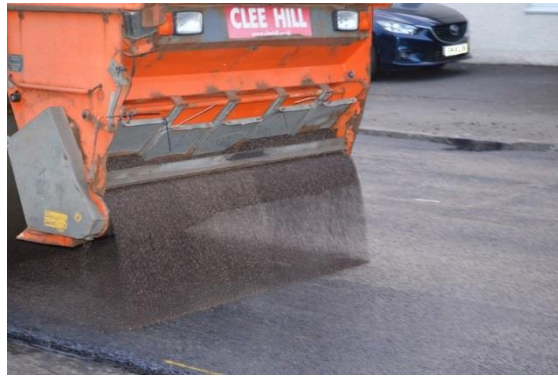
Figure 2-3 Surface gritting application from steel drum roller
