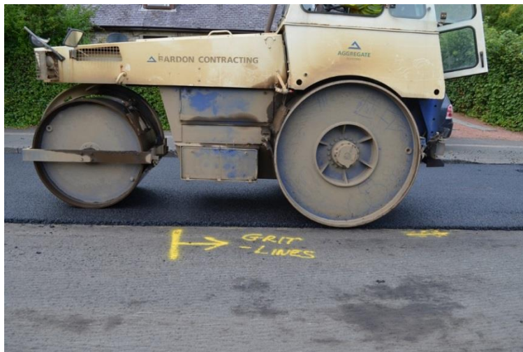
Figure C-4 Compaction of surface course by Aggregate Industries
