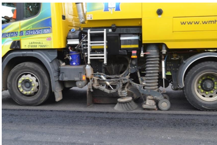
Figure C-3 Sweeping of the longitudinal joint
