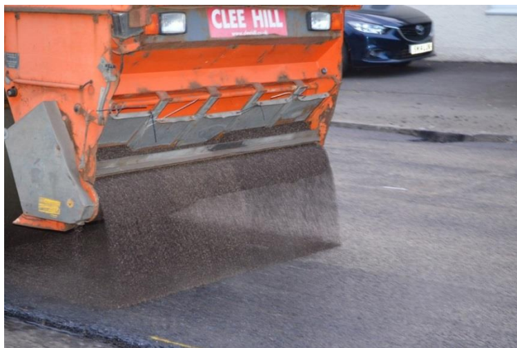
Figure C-6 Gritting prior to line marking
