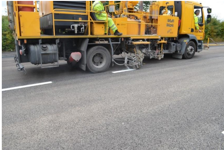
Figure C-7 Drying/Blowing prior to line marking application
