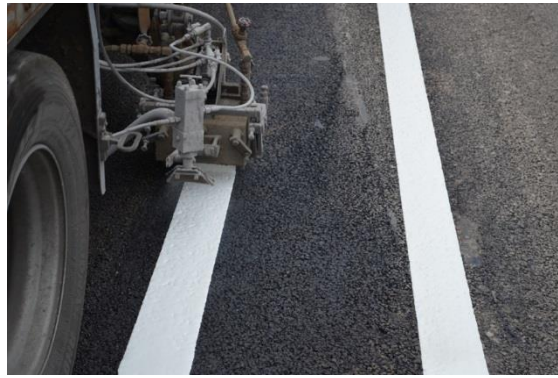
Figure 2-5 Road Marking application
