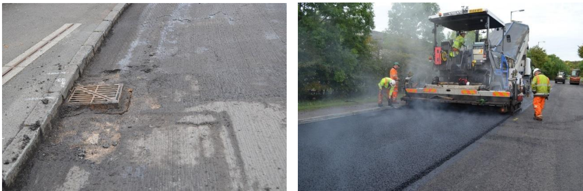
Figure 2-1 Asphalt laying operation (left - milled surface, right – laying of surface course)
