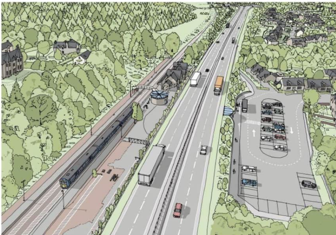
Illustration 7.7. An artist's impression showing an at-grade A9 carriageway and the replacement car parking facility at Birnam Industrial Estate
