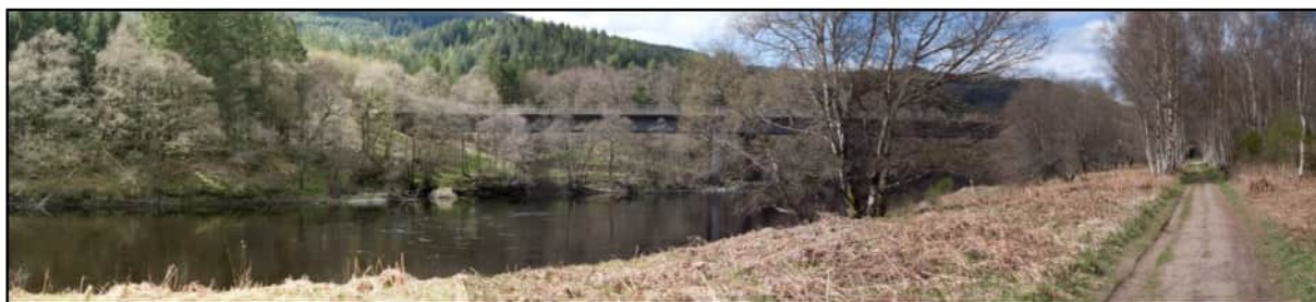
Photograph 13.4: View looking north-west towards the existing A9 from NCR77, south of the Tay Crossing (Viewpoint 17)
