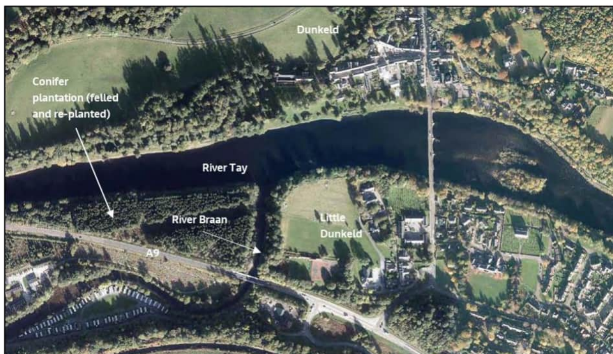
Image 12.1: Aerial photograph of Dunkeld, Dunkeld Bridge, Little Dunkeld, the River Braan crossing and A9 road corridor at the existing Dunkeld Junction
