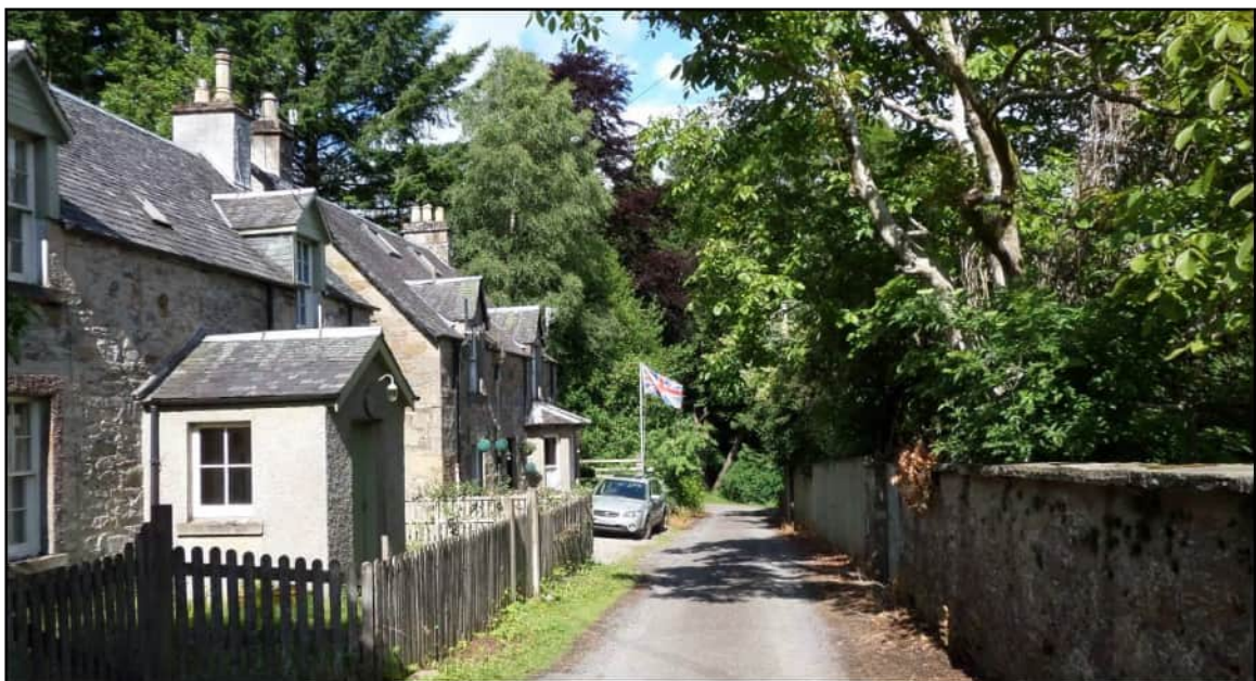
Photograph 14.5: Elsey Cottage and Birnam Bank Cottage (Assets 17 and 18), Category C Listed Buildings, within Birnam Conservation Area (Asset 44), July 2015
