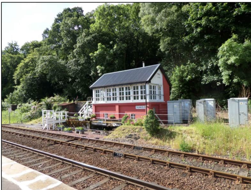
Photograph 14.4: North-east facing elevation of Dunkeld and Birnam Station Signal Box (Asset 16), a Category B Listed Building, facing south-east
