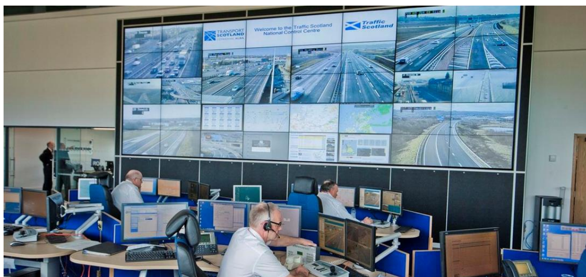
Photo 6.4: Traffic Scotland National Control Centre – Control Room
