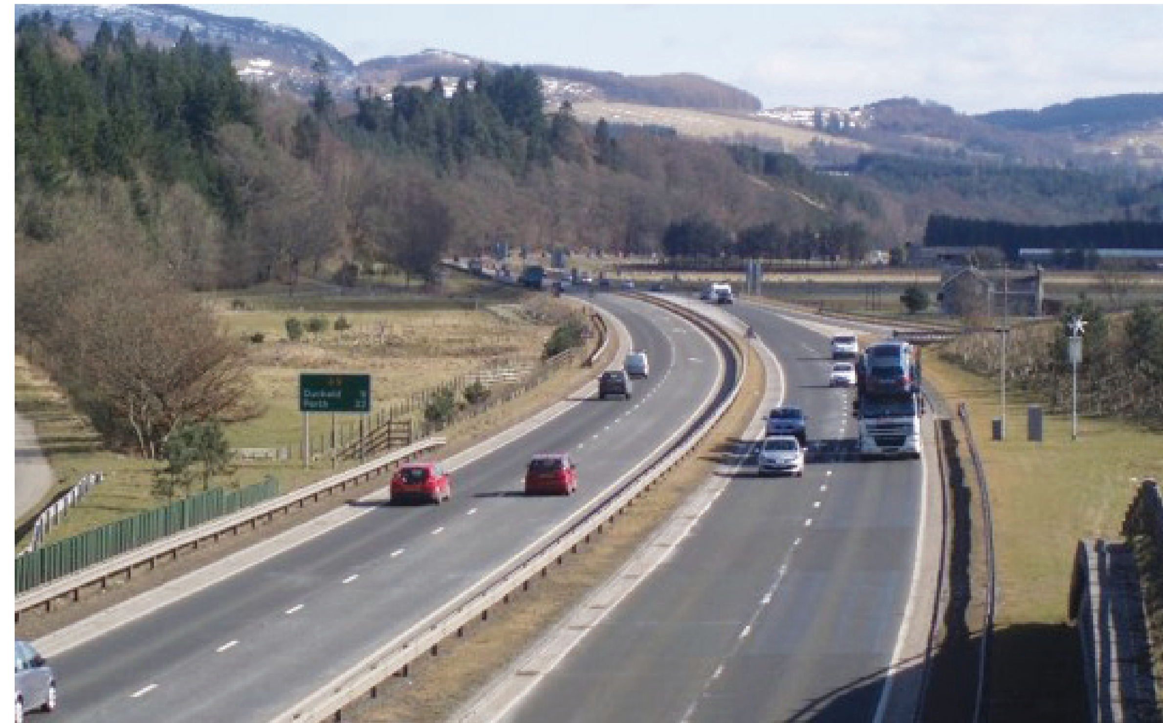
View of existing dualled section from Ballinluig Junction looking south
