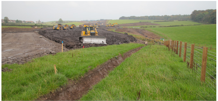
Earthworks embankment construction – Glasgow-Ayr railway line to Blair Road
