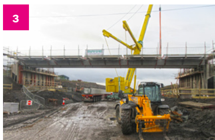
1 - 2. Construction of the abutment bases and walls for the Blair Road Bridge; 3. Edge beam being lifted into position; 4. Test Pile being installed at the River Garnock Viaduct
