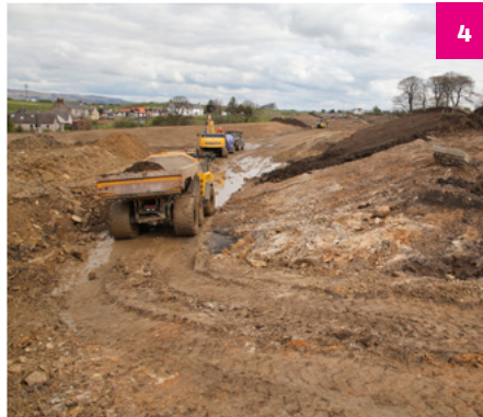
1. Viaduct structure launch platform being constructed in preparation for the delivery of the steel girders; 2. Reinforcement cage for the column foundations being installed adjacent to the River Garnock; 3. Embankment slope with the new Blair Road overbridge in the background; 4. Topsoiling of the embankment slope at Highfield; 5. Cattle underpass installed at the eastern end of the project
