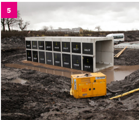
1. Viaduct structure launch platform being constructed in preparation for the delivery of the steel girders; 2. Reinforcement cage for the column foundations being installed adjacent to the River Garnock; 3. Embankment slope with the new Blair Road overbridge in the background; 4. Topsoiling of the embankment slope at Highfield; 5. Cattle underpass installed at the eastern end of the project
