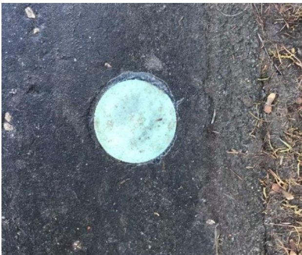
Figure 6-5 Protruding From Surface
