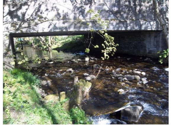
Photograph 9b: Typical channel cross-section downstream of the existing A9 (looking downstream)
