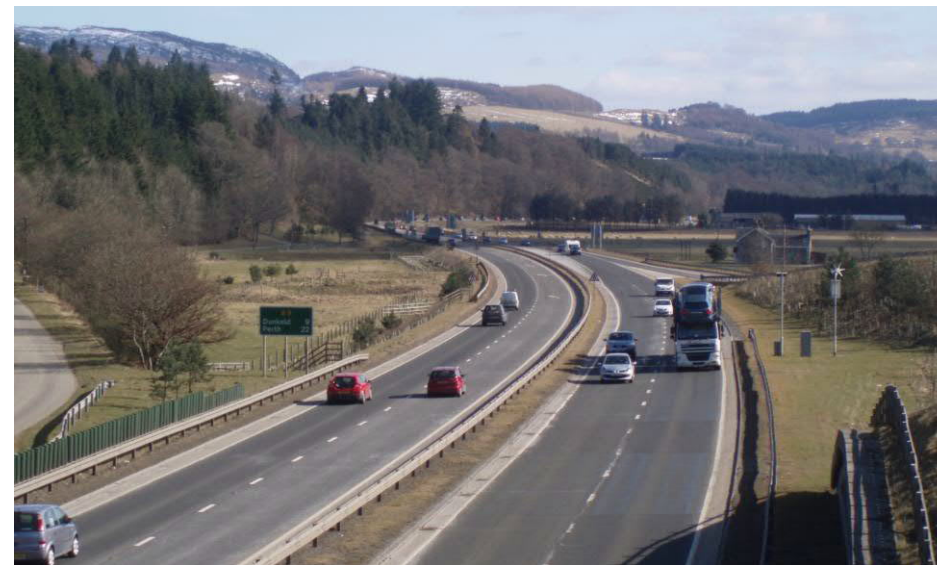
Photograph 1: View of the existing dualled section near Ballinluig, looking south
