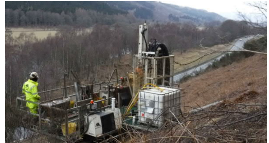
Photograph 10: Ground investigation works for the proposed scheme
