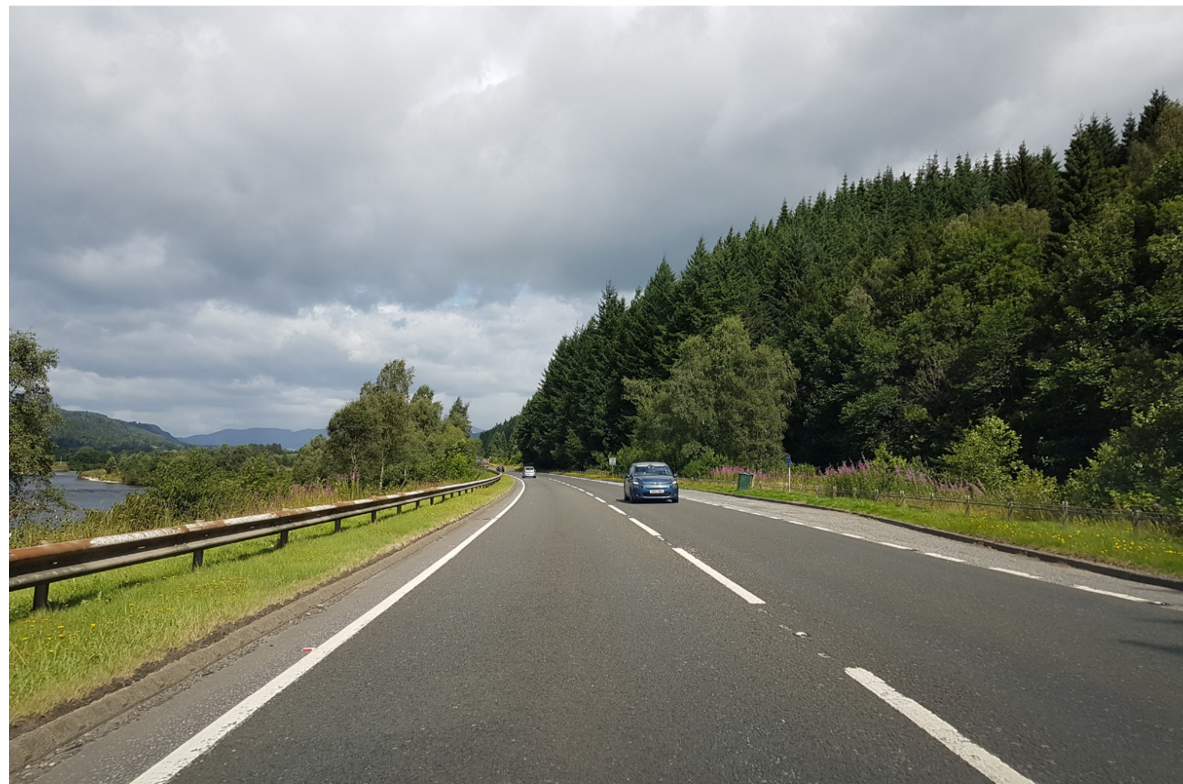
View of the A9 at the southern extents of the scheme, looking north
