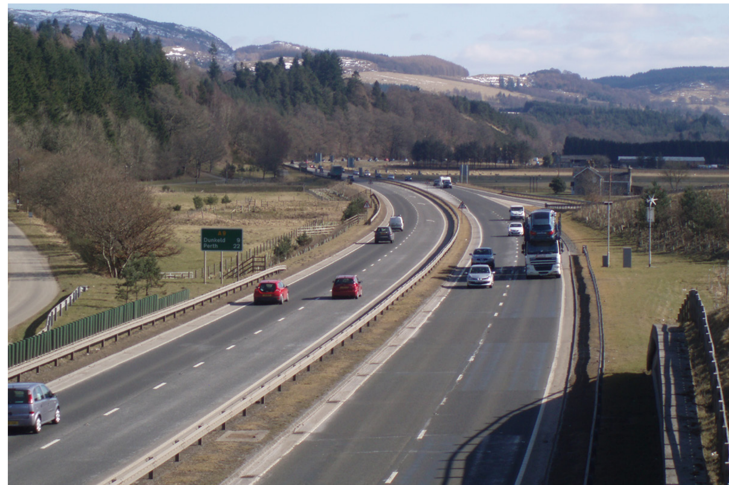
View of the existing dualled section near Ballinluig, looking south
