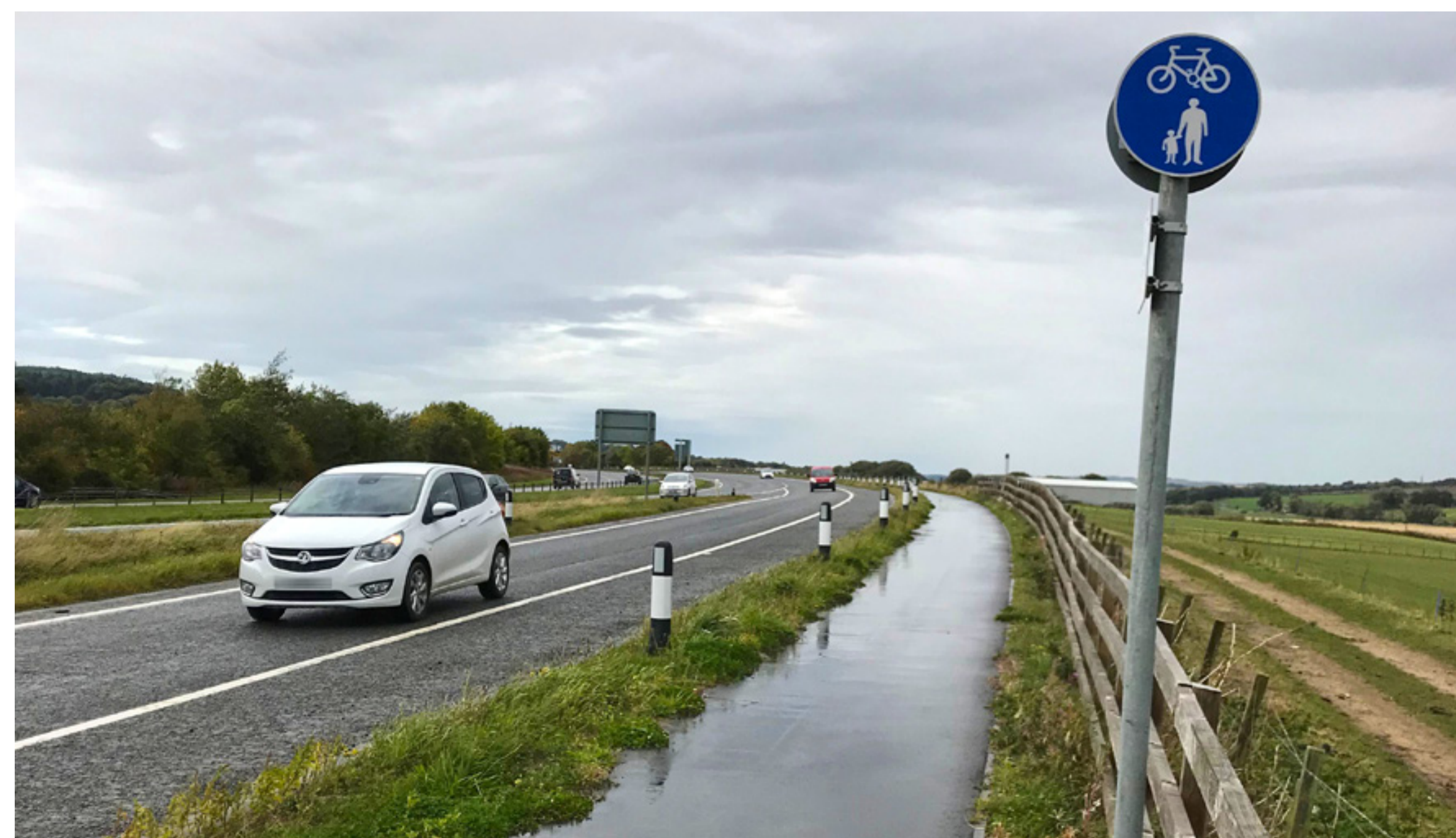
Existing footway/cycleway facility at A96 Tavelty junction
