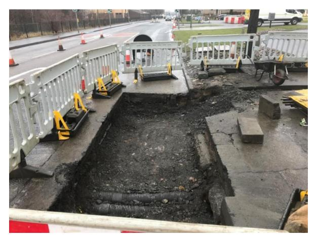
Figure 2 - Traditional trench methods showing a large exposed area
