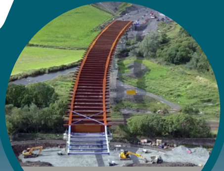
River Garnock Viaduct
