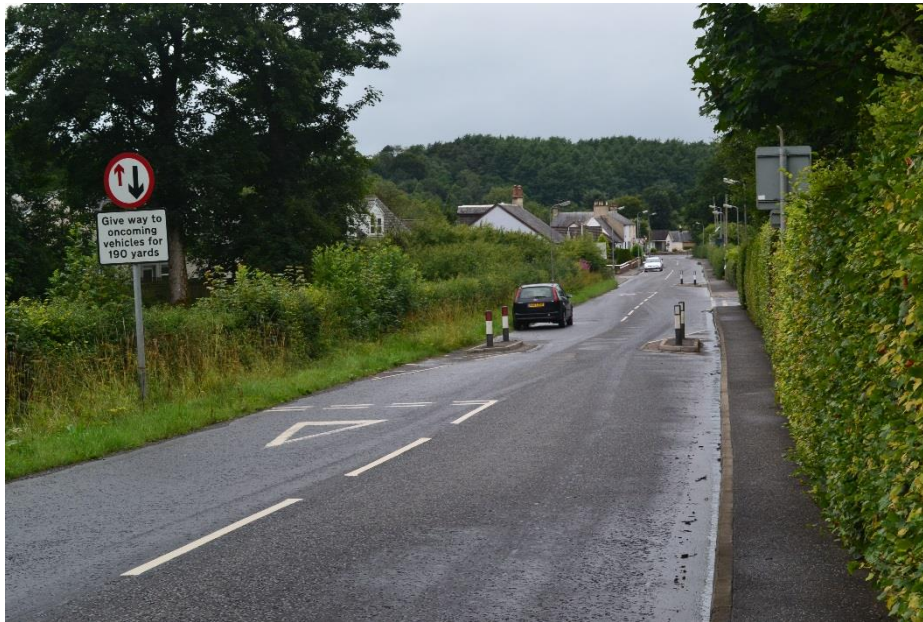
Figure 2-2 B473 Sorn: buildouts with priority working
