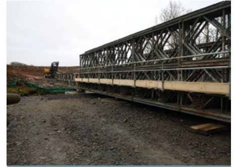
Bailey bridge with 'launching nose' attached at the Shochie Burn
