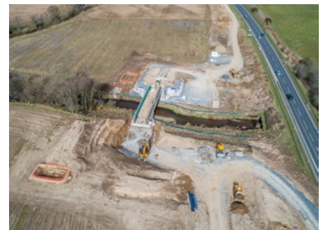
Bailey bridge in its final position at the Ordie Burn
