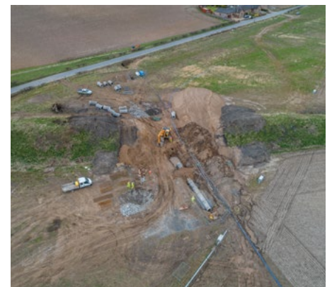
Drainage culvert installation Stanley Road
