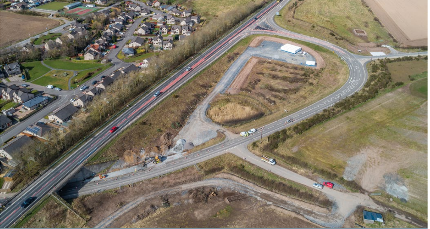
Construction underway to extend at Hunters Lodge Underbridge
