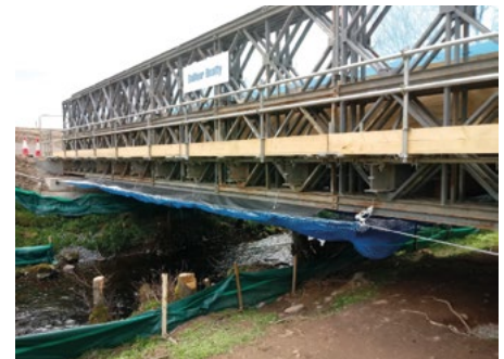
The catch net prevents debris from landing in the burn below
