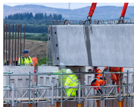
Precast beams being lifted into place
