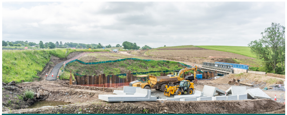
Culvert extension at the Shochie Burn
