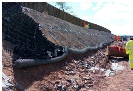
Soil nailing works
