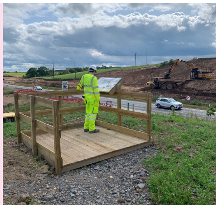
Viewing platform adjacent to the Pitlandie overbridge
