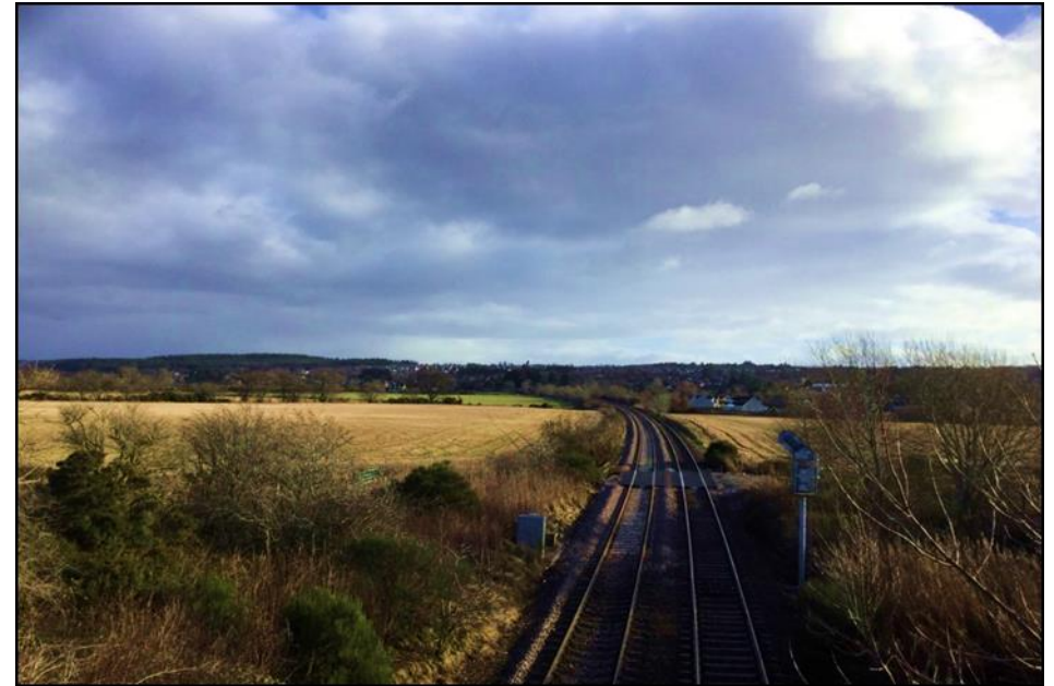
Photograph 1: Highland Main Line Railway looking east from the existing NMU crossing
