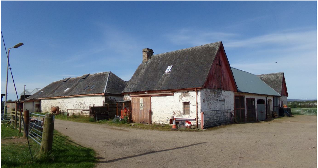
Photograph 14.3: Single-storey Agricultural Ranges Forming part of Ashton Farm (Asset 18), Facing West
