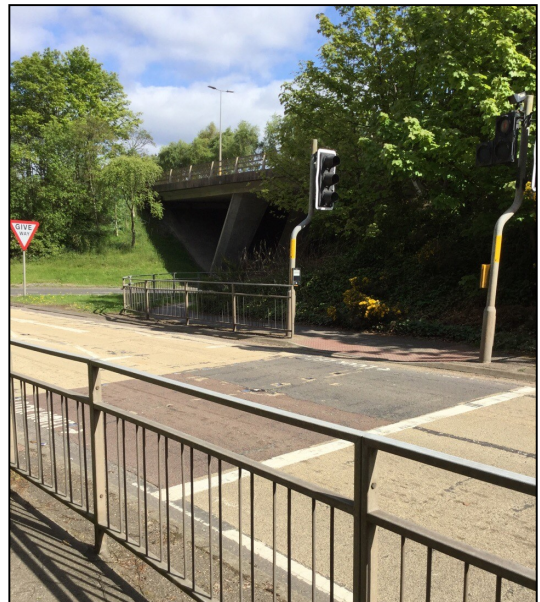
Photo 16.11: Crossing of the A9 at the Raigmore Interchange connecting LP9 and IN19.16
