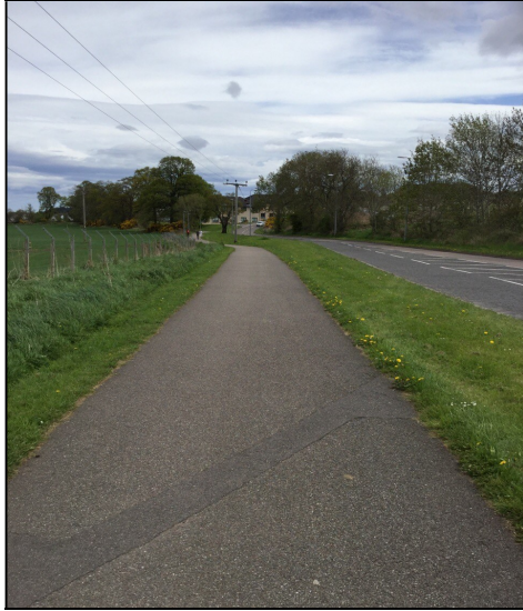
Photograph 16.12: Section of the NCN 1 on U1058 Caulfield Road North
