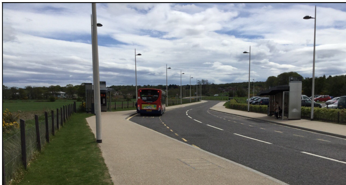
Photograph 16.13: Two Bus stops on the Inverness Campus Access Road (LP2)
