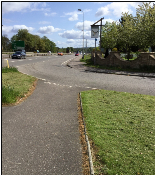
Photograph 16.10: LP9 looking north on the A96 Carriageway
