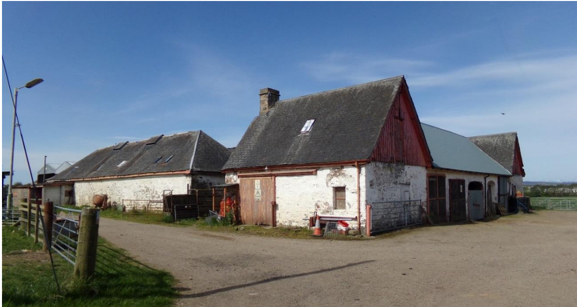
Photograph A14.5: Single-storey agricultural ranges of Ashton Farm (Asset 18), facing west
