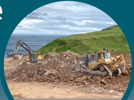
Rock excavation work
