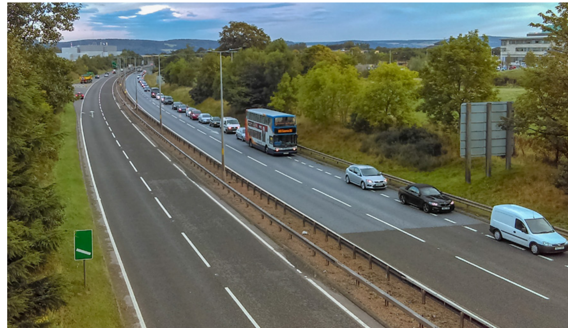
Existing A9 Southbound Inshes Junction diverge (looking north)
