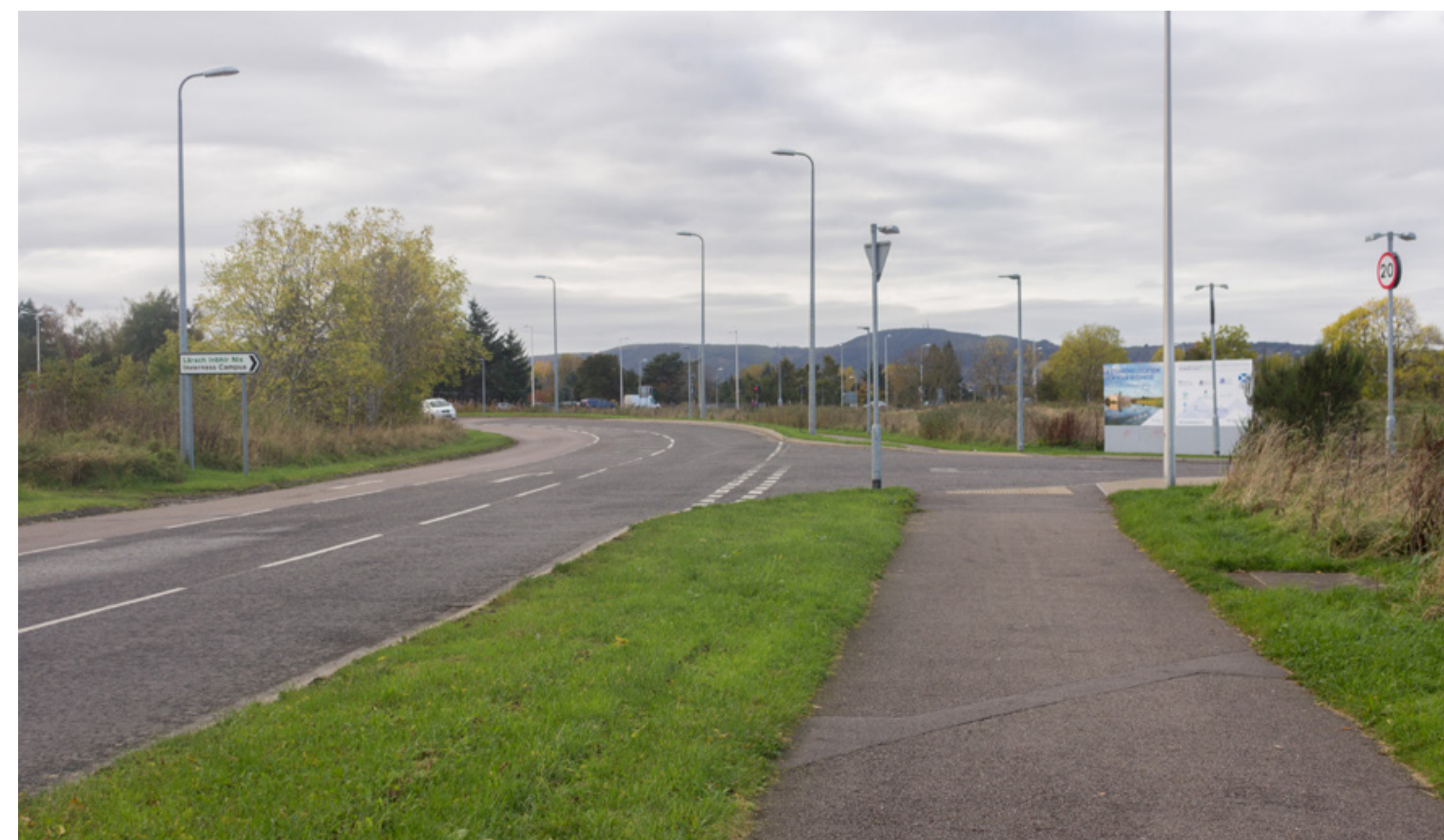
Existing Caufield Road North (looking north)
