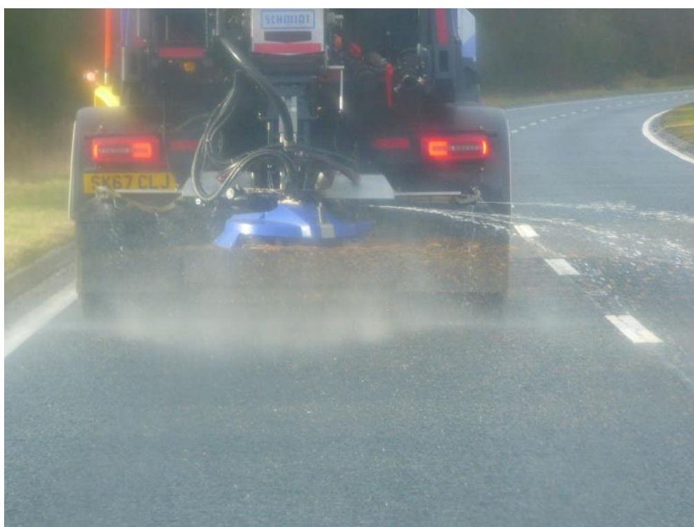
Figure 10. Spreading of high brine share pre-wetted salt.
