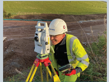
Elliot Moir setting out at the new Stanley/Tullybelton junction
