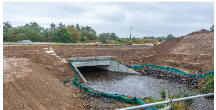
Ordie culvert extension
