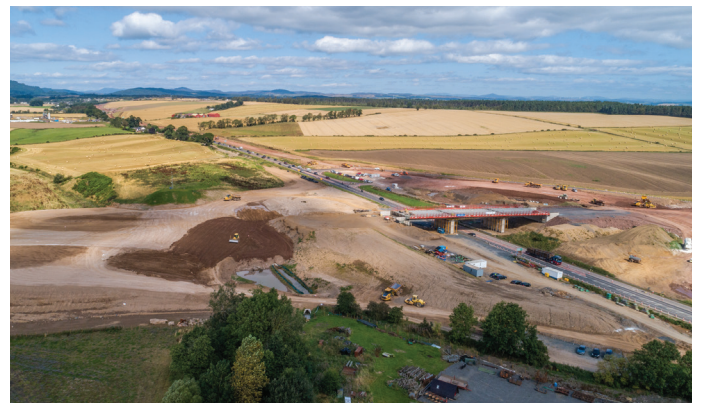
Progress at the Stanley/Tullybelton junction
