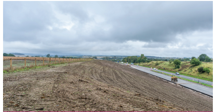
New embankment and carriageway preparation at Luncarty
