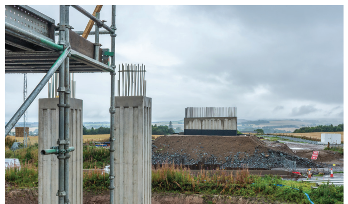
Columns under construction at Coltrannie
