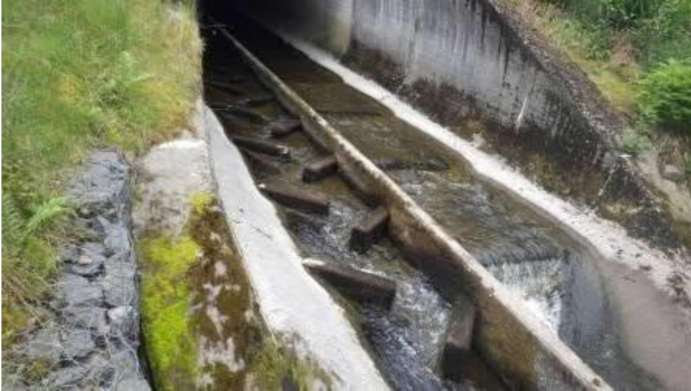
Figure 36. Downstream outlet of FB21394.
