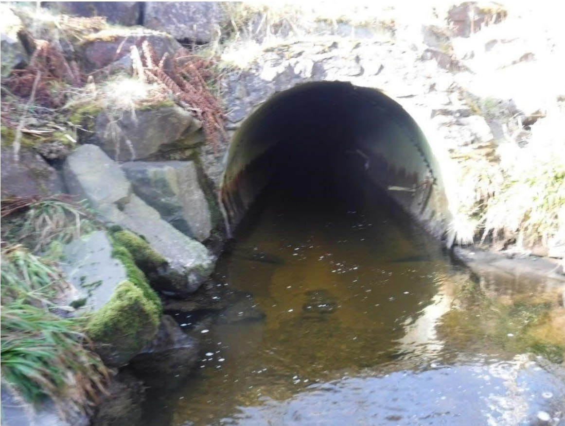
Figure 34. Downstream outlet of FB1423.
