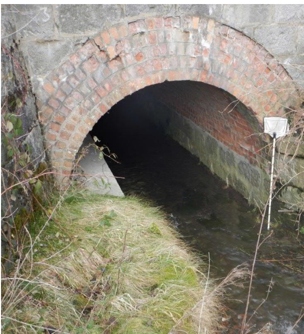
Figure 31. Upstream inlet of Culvert 3.
