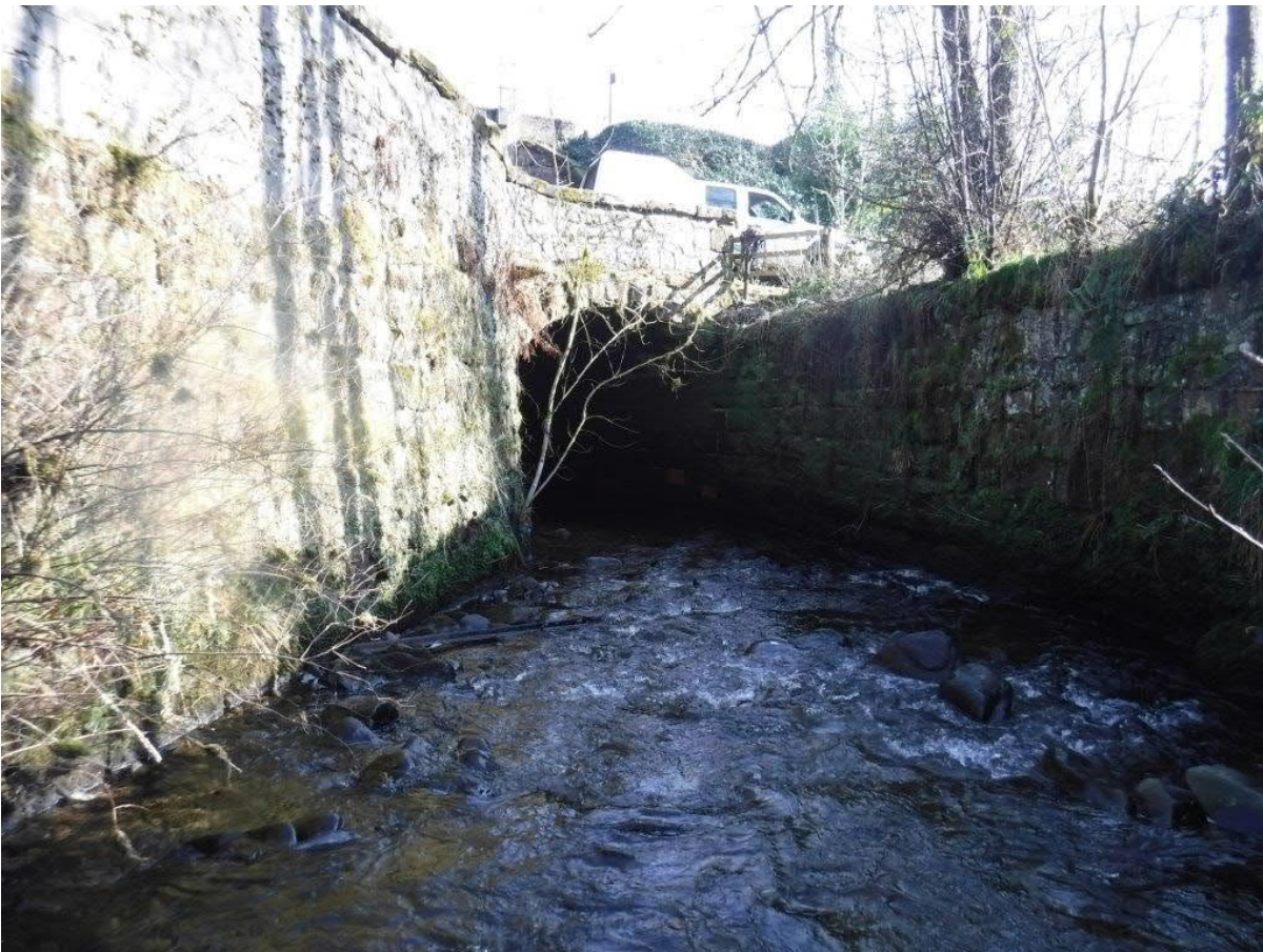
Figure 33. Upstream inlet of FB1423.
