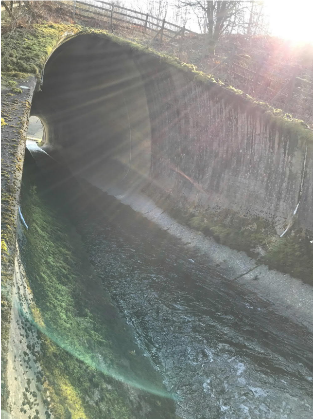
Figure 35. Downstream outlet of FB1424.
