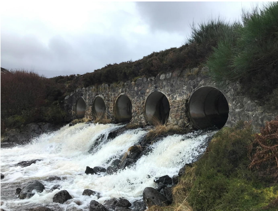
Figure 32. Downstream outlet of FB602.
