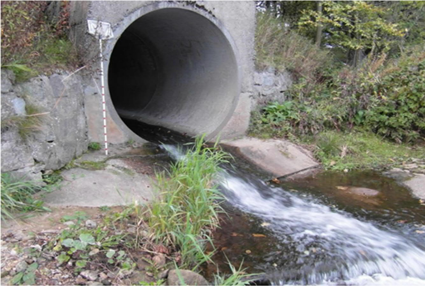
Figure 26. The downstream outlet of FB20689.
