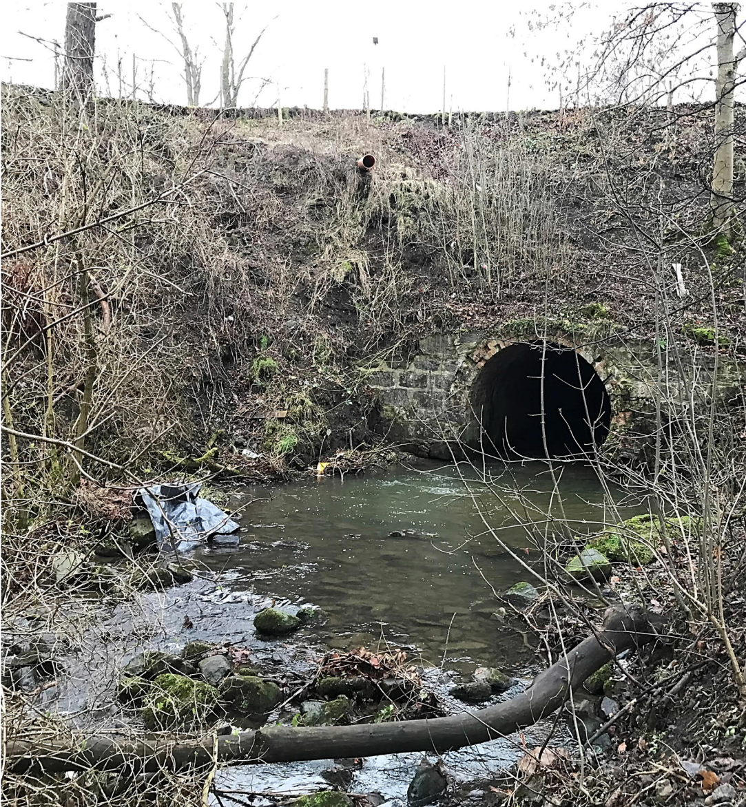
Figure 27. The downstream outlet of FB20690.
