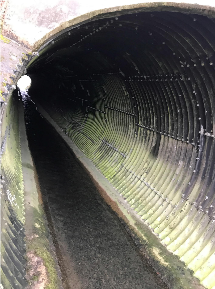
Figure 28. View from the outlet facing upstream (FB3176).
