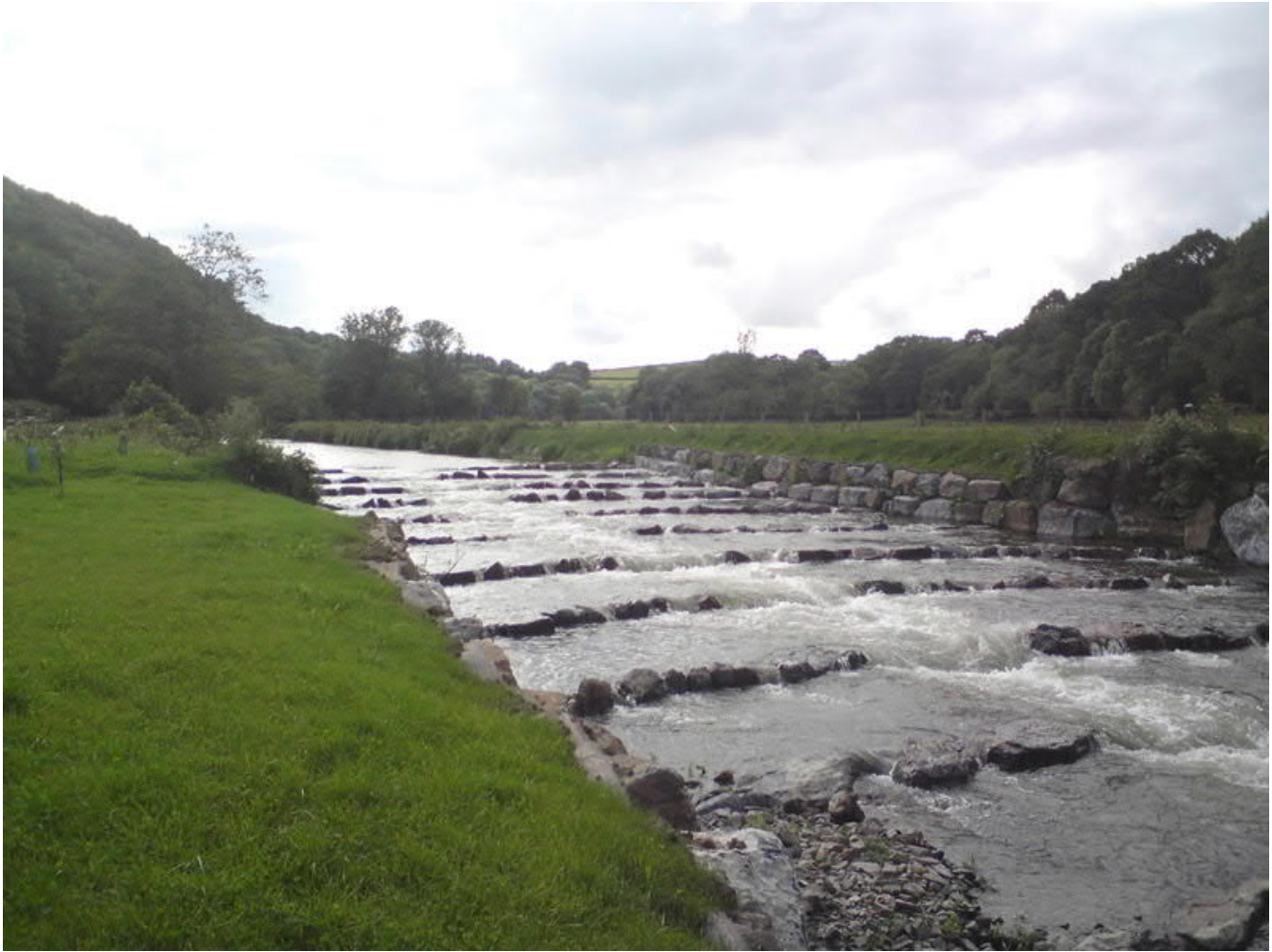
Figure 15. Photograph of the finished fish pass.
