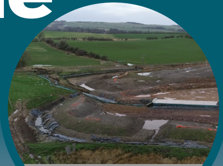
The culvert under construction at Smithston
