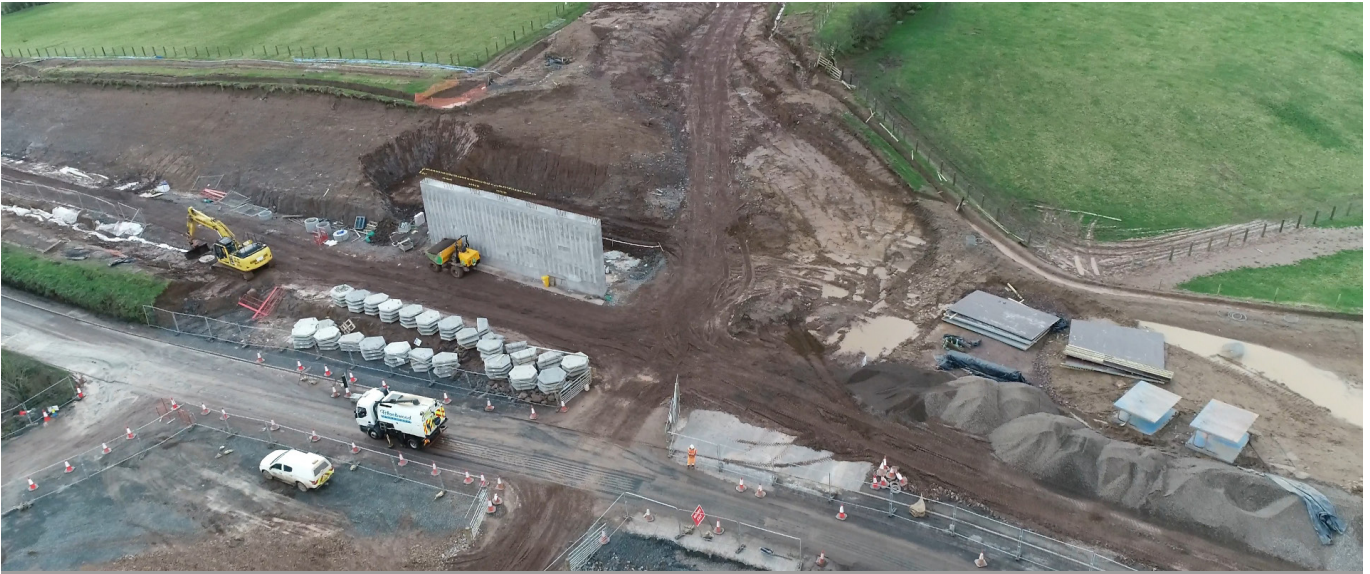
Alloway Road Underpass under construction
