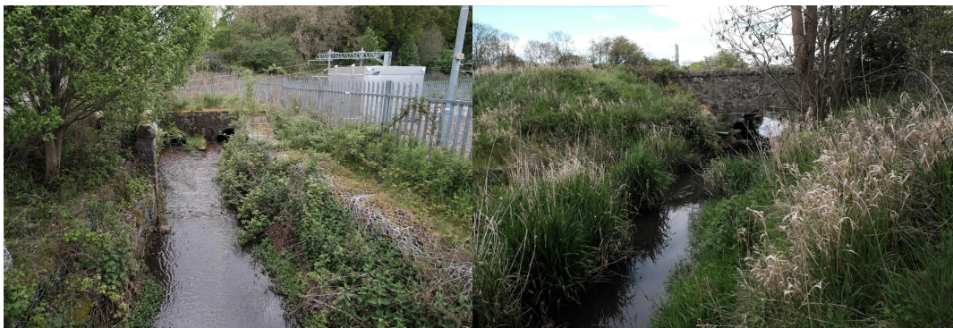
Figure 2-6 Swine Burn channel downstream of syphon and downstream of unnamed bridge 2 showing long grass along banks and straight channel.
