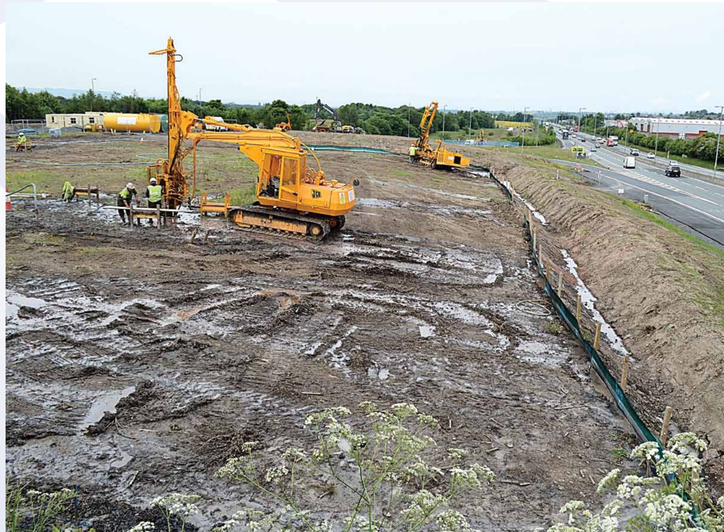
Advance works got underway earlier this year.
