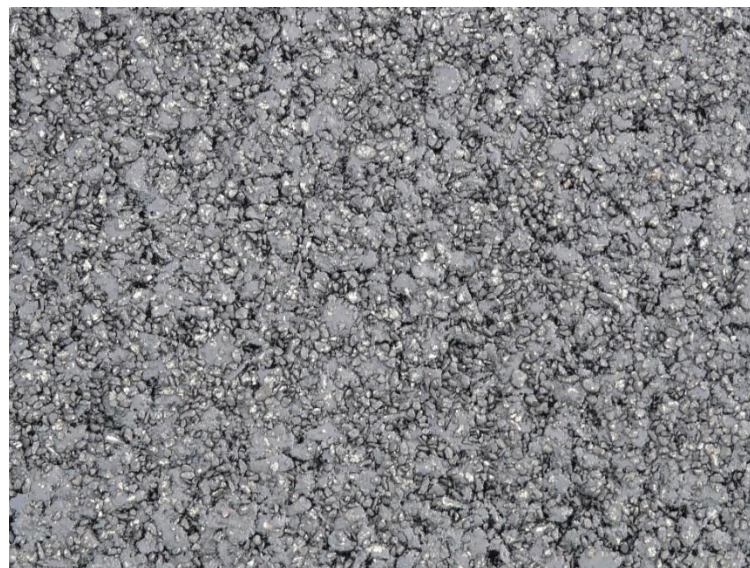
Figure 2-3 - New TS2010 surface course after gritting (TRL670)
