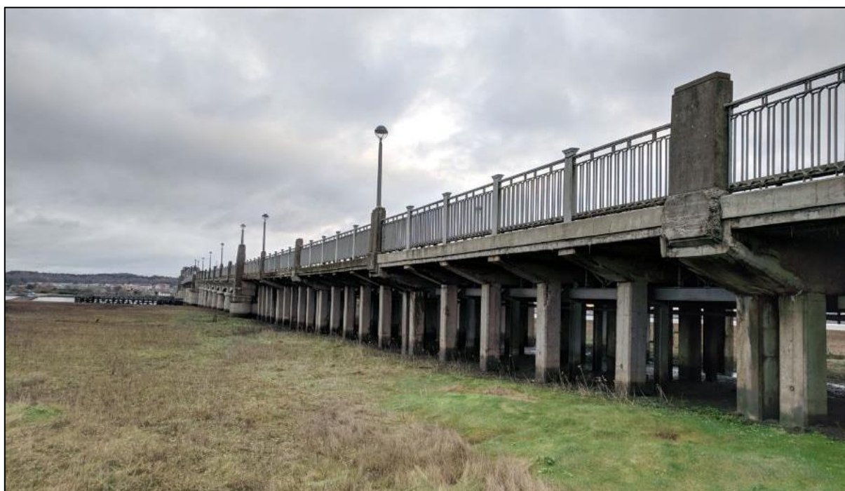
Photograph 1: Kincardine Bridge (Showing Existing Piled Viaduct)
