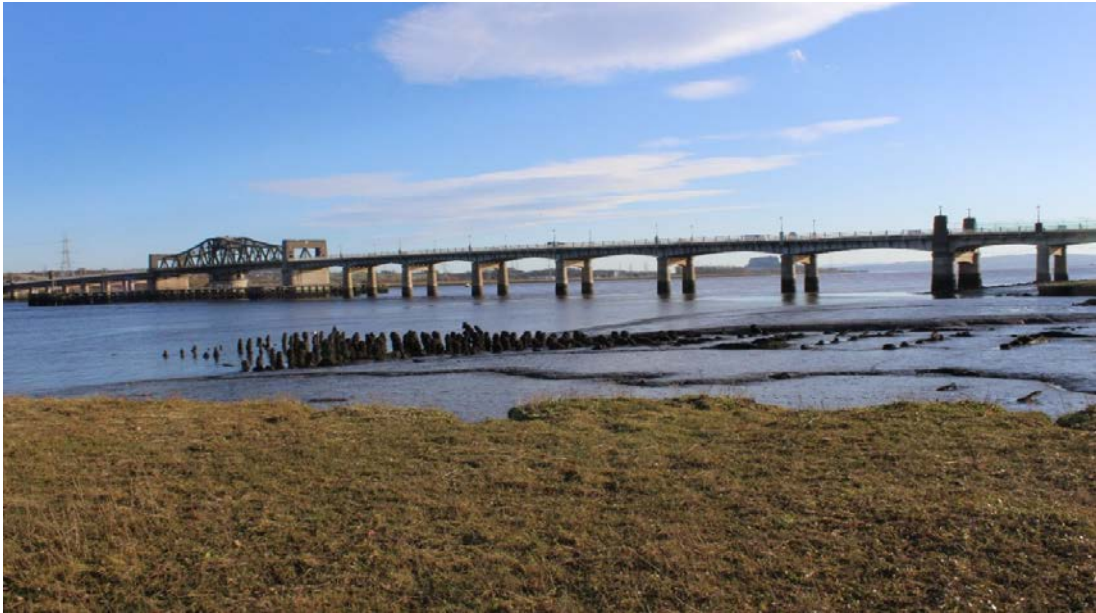
Photograph 10.3: Higgins' Neuck Ferry Pier (Asset 14), looking south-east
