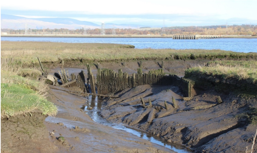
Photograph 10.1: Higgins' Neuck Landing Point (Asset 11) and associated timber-lined sluice, looking north-east
