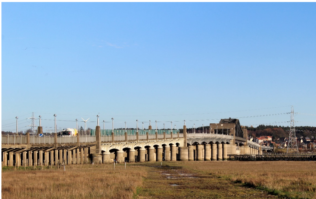
Photograph 10.5: the Kincardine Bridge (Asset 15), looking north-east
