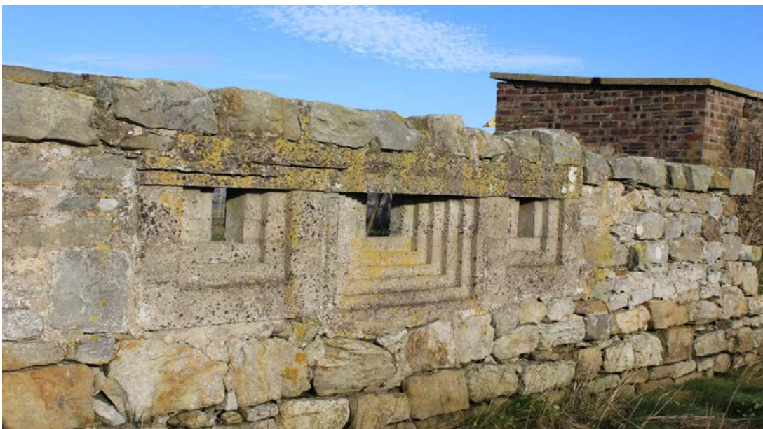
Photograph 10.4: Higgins' Neuck Machine Gun Post (Asset 12), looking north
