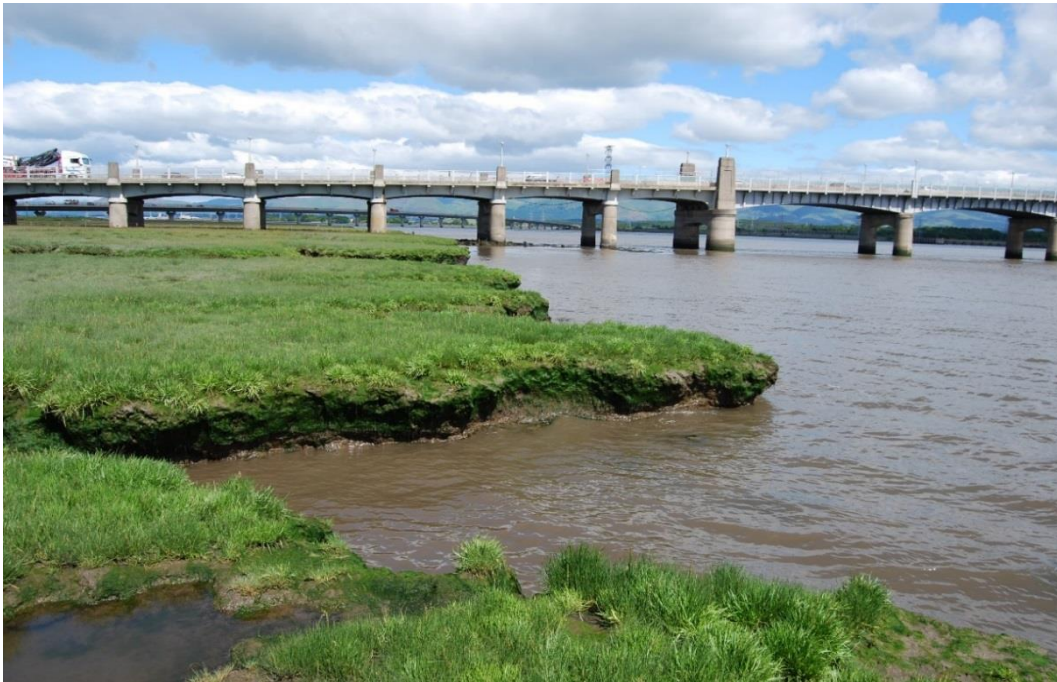
Photograph 4: View of Marsh Edge on Downstream Side of Kincardine Bridge
