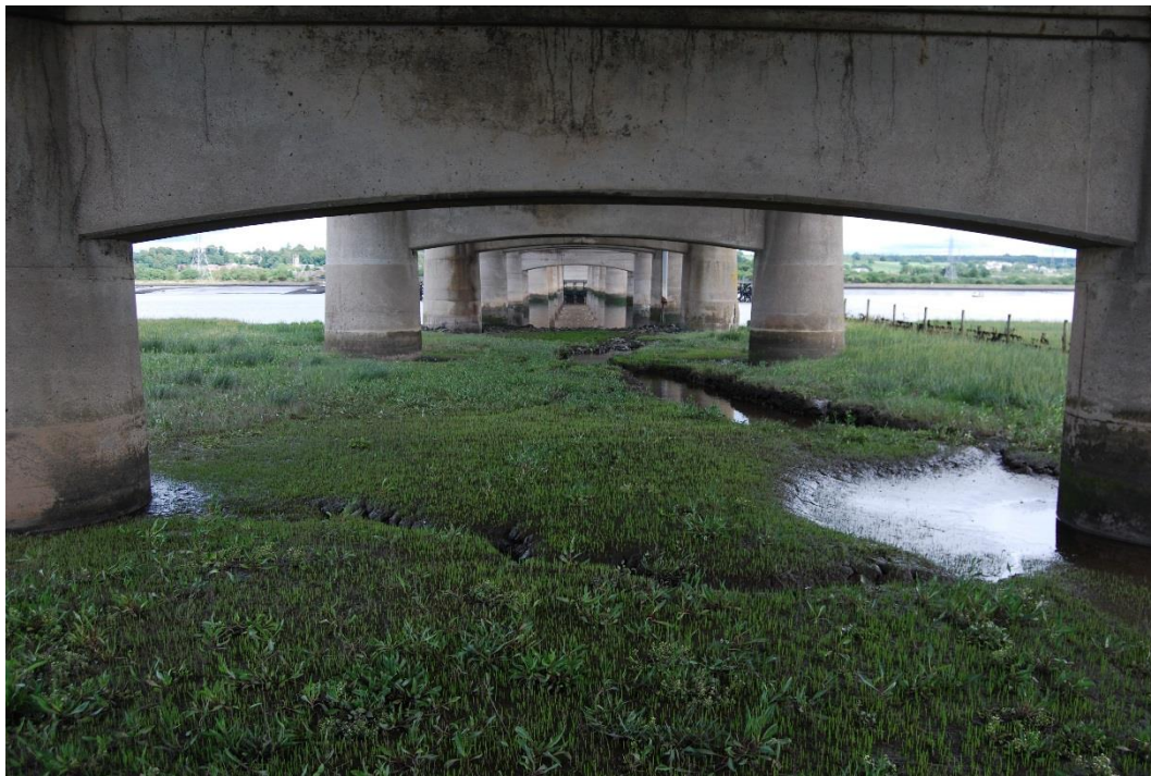
Photograph 7: Glasswort Vegetation with Sea Aster under the Existing Viaduct
