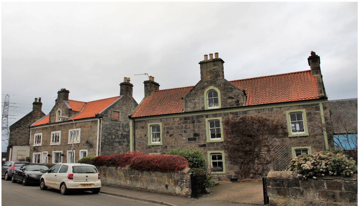
Photograph 8: Numbers 26, 28 and 30 Keith Street Kincardine-On-Forth (Asset 18) on the right; and 34 and 36 Keith Street (Asset 17) on the left, looking north-west
