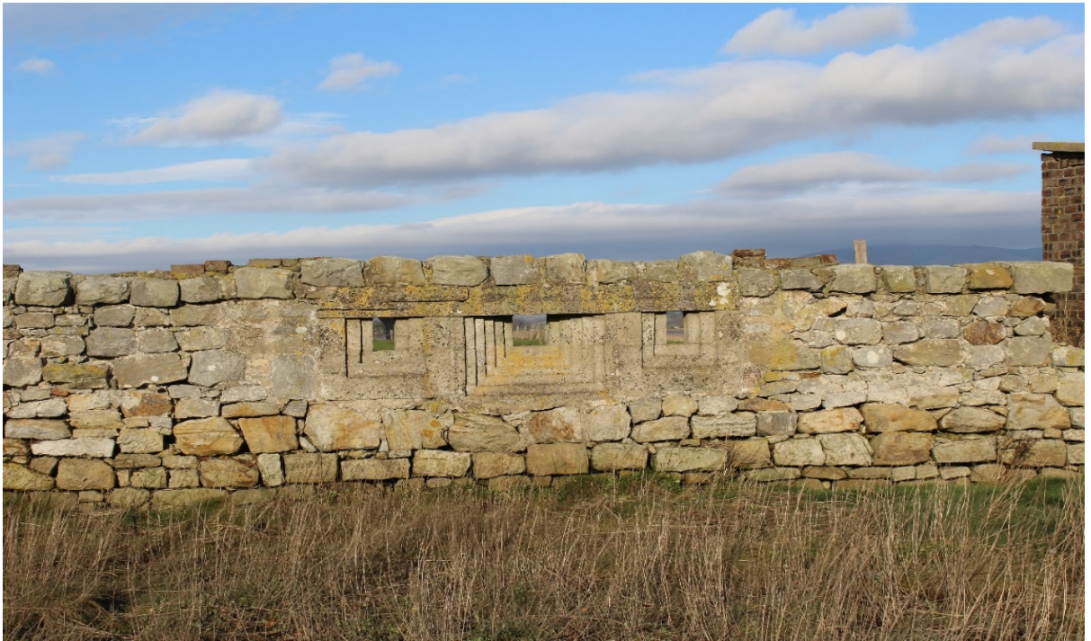
Photograph 4: Higgins' Neuck Machine Gun Post (Asset 12), looking north
