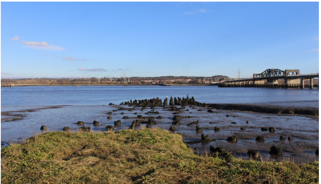
Photograph 2: Higgins' Neuck Ferry Pier (Asset 14) with view to the corresponding ferry pier at Kincardine, looking north-east
