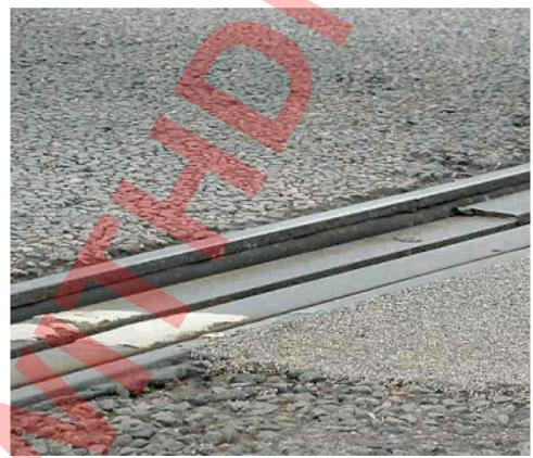
Figure 8 Viaduct (Insitu concrete deck) Built 1986 [Damage to the West Deck Expansion Joint- Rail broken in the middle and level difference.]
