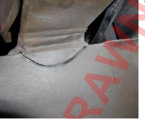
**Figure 3** Cable Stayed Bridge (Composite steel-concrete deck) Built 1991 [Fracture in the support joist immediately below the welded connection to the rail.]
