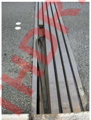
Figure 2 Viaduct (Precast Prestressed Concrete) built in 1993 [The damaged rail has been taken out of the joint and corrosion is visible on the rails.]
