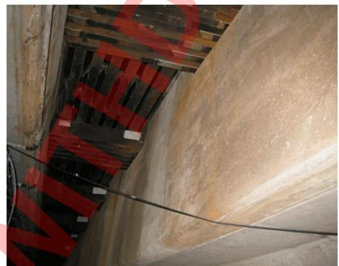
Figure 4 Cable Stayed Bridge (Composite steel-concrete deck) Built 1991 [Rust staining from expansion joints over pier (Seal replacement stopped water ingress.]
