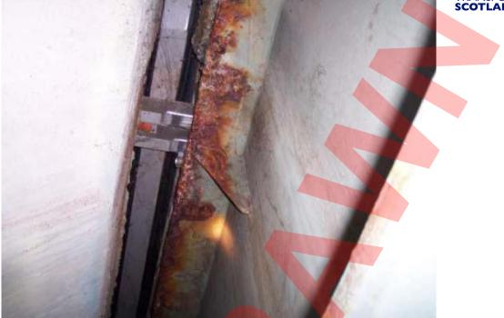
Figure 7 Viaduct (Precast Prestressed Concrete) Built 1976 [Failure of joint on footway. Seal failed between rails on carriageway.]
