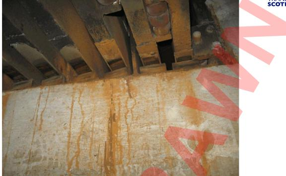
Figure 5 Cable Stayed Bridge (Composite steel-concrete deck) Built 1991 [ Corrosion to expansion joints sliding plates over pier.]
