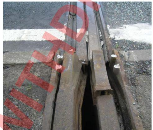
Figure 6 Cable Stayed Bridge (Composite steel-concrete deck) Built 1991 [Trimmer Beam Support Steelwork corroded.]
