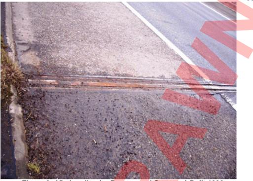
Figure 9 Viaduct (In-situ Prestressed Concrete) Built 1990 [ Corrosion to rails and debris in seals.]
