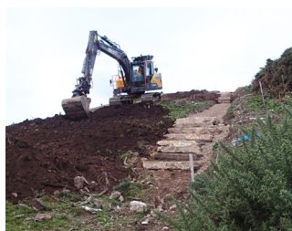
Installing stone steps at John O'Groats trail
