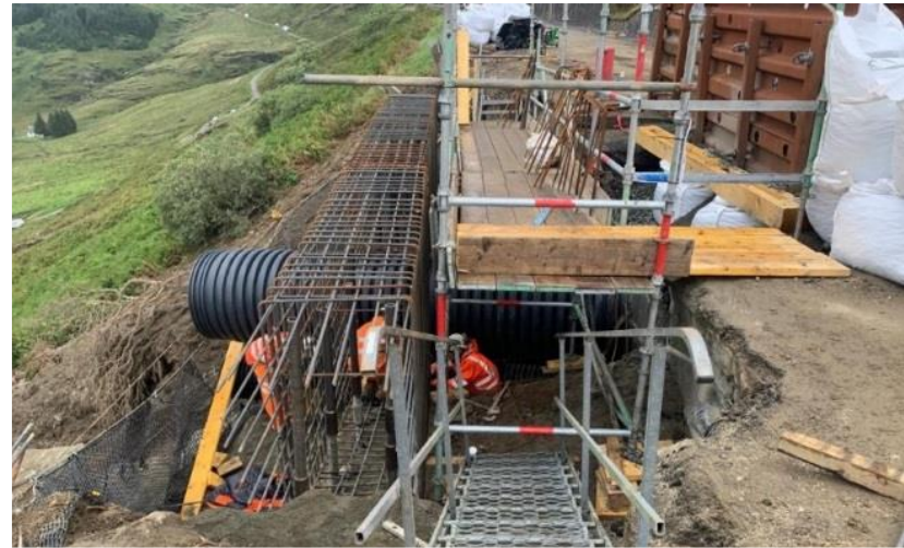
Construction of new retaining wall/culvert
