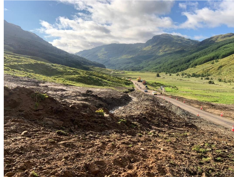
Enhanced earthwork bund enhanced above Old Military Road.
