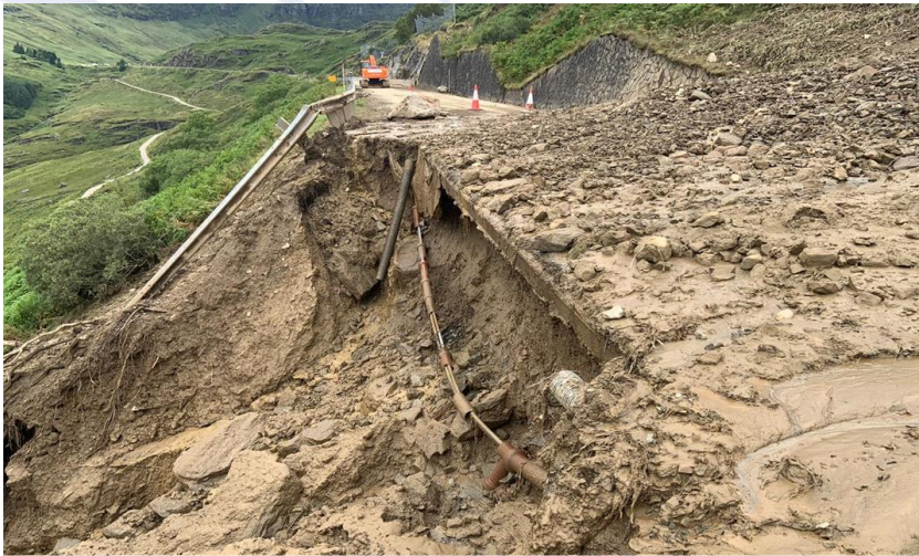
A83 carriageway inundated and undermined
