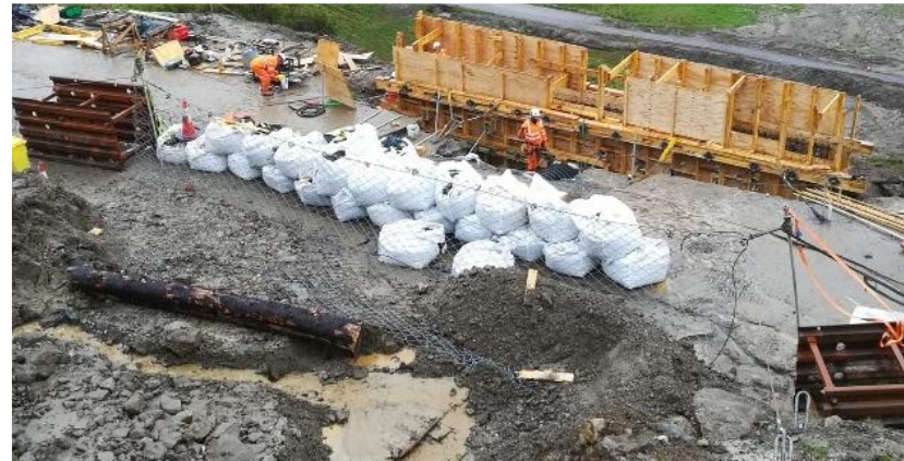
Temporary pit and roadside mitigation
